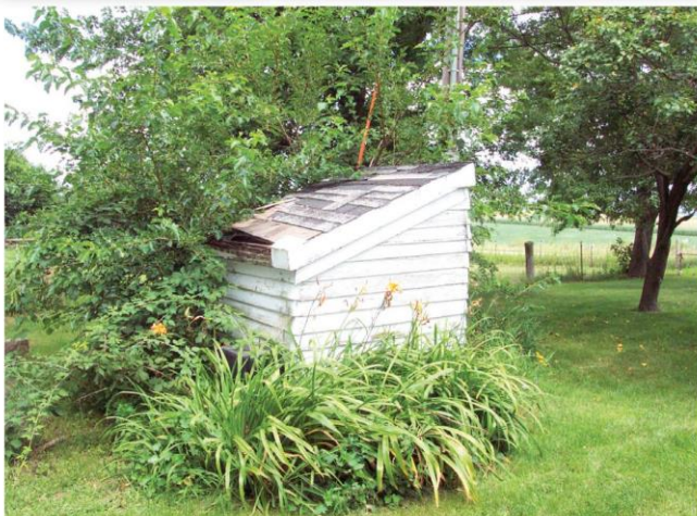
Examples of wells that should be plugged.
