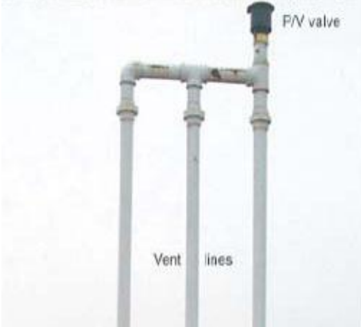
Three vent lines manifolded into one.
