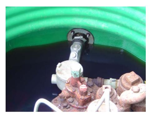
This photo shows product released up to the penetration seal of an STP sump (electrical conduit). If these seals are not tight, a release can occur, or product and vapors can travel through the pathway. The problem here was in the primary wall of the piping. The sump did its job and the test boots were open to allow product to flow into the sump. Although this leak should have been detected a lot earlier.
