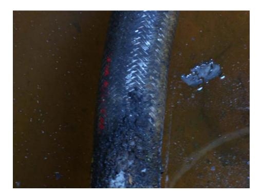
Deteriorated and leaking flex connector sitting in product and water. Flex connectors must be isolated from water and backfill (or protected).
