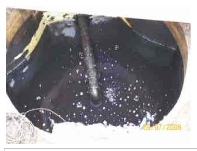
One of our compliance inspectors discovered this uncontained sump full of diesel fuel. After the pressurized system was activated, bubbles came up from the backfill. An unprotected flex connector was corroded and the site will undergo an expensive cleanup. The inspector told the operator to take the tank out of service and to report it to the DNR.
