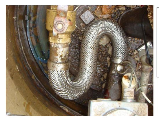
These are severe bends in a flex connector-beyond what is recommended by the manufacturer. A rupture and leak will eventually occur.
