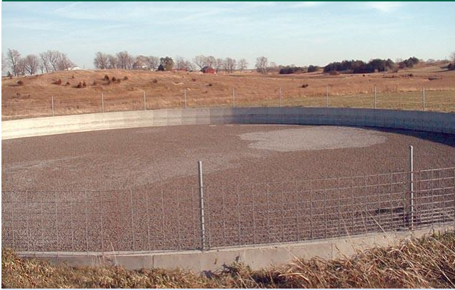
Liquid swine manure in concrete pit covered with Leka rock.
