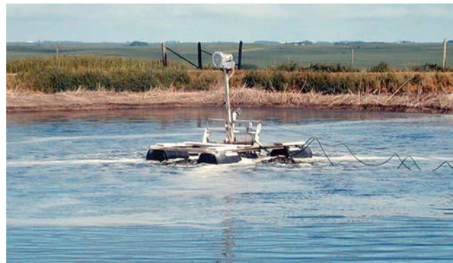
Aerator on second-stage lagoon at swine facility will reduce hydrogen sulfide emissions, but may also increase ammonia emissions.
