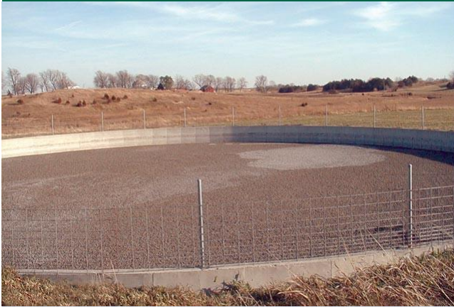
Liquid swine manure in concrete pit covered with Leka rock.
