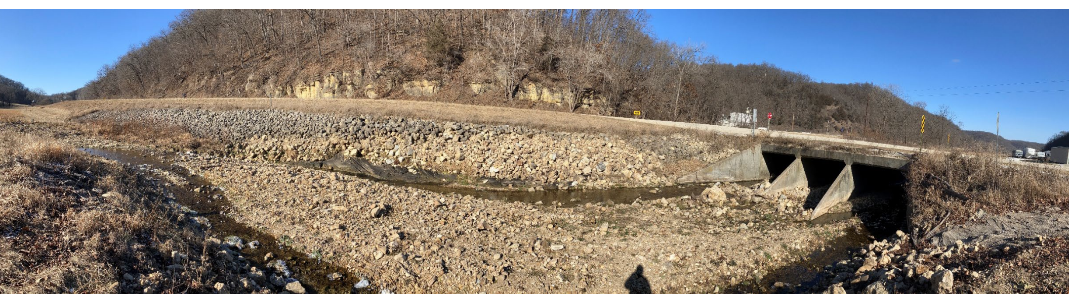
Photo looking north at Site 2 along Clear Creek at approximately 170 linear feet of proposed bank stabilization work. 01/13/2025
