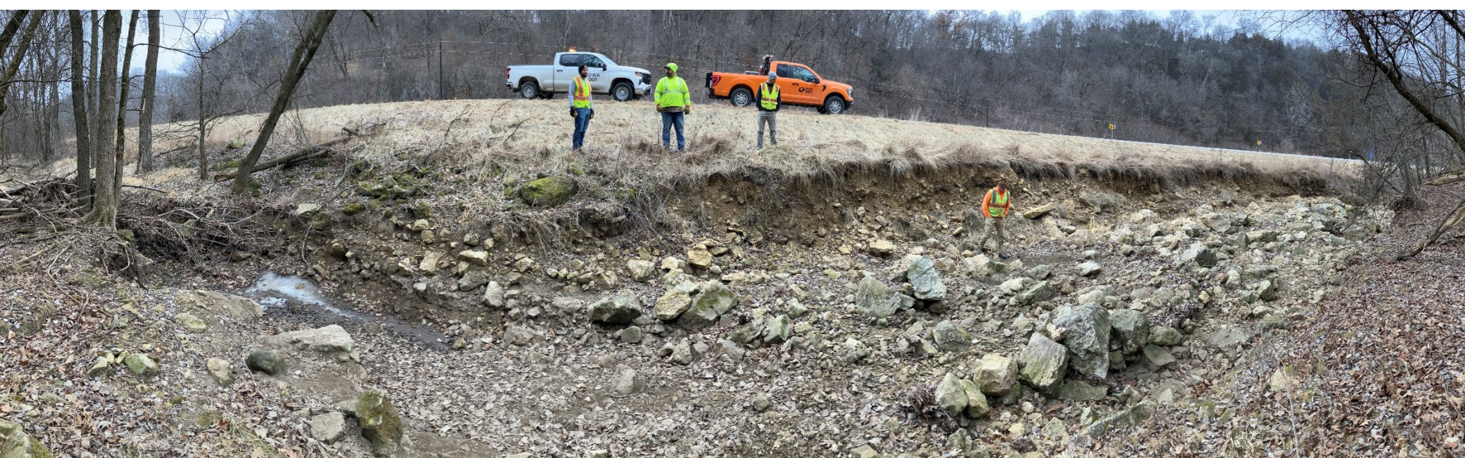
Photo looking north at Site 1B along Clear Creek at approximately 466 linear feet of proposed bank stabilization work. 02/03/2025
