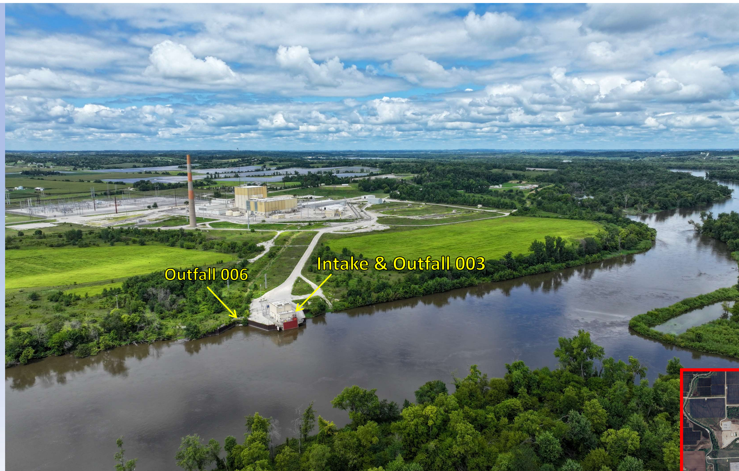
Intake and Discharge Structures
