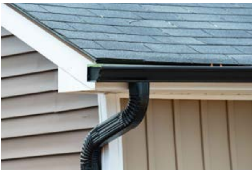
Asphalt shingle collection surface. Image courtesy of Google images.
