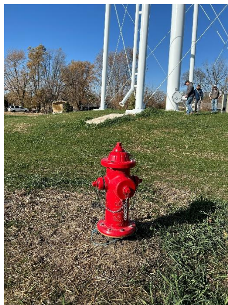
New hydrant installed in conjunction with a new elevated storage tank.
