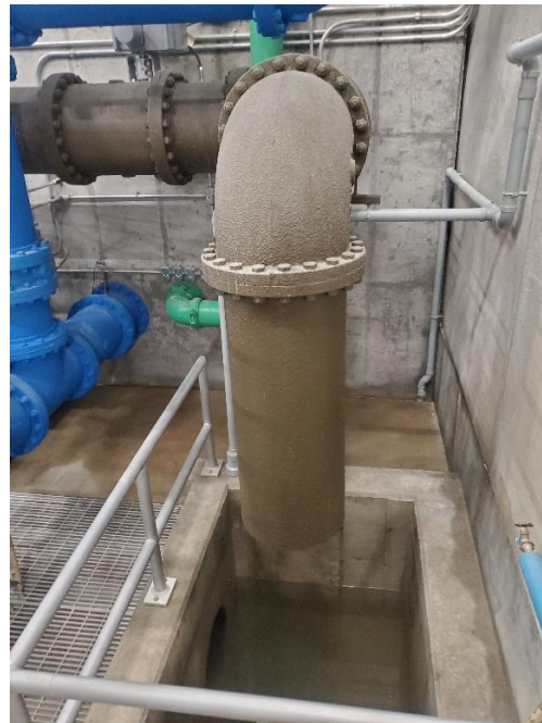
Wastewater collection in the filter pipe gallery of a new surface water treatment plant, constructed primarily in 2025 using DWSRF funds. Filter effluent diversion to waste is shown on the left and backwash water collection is shown on the right.
