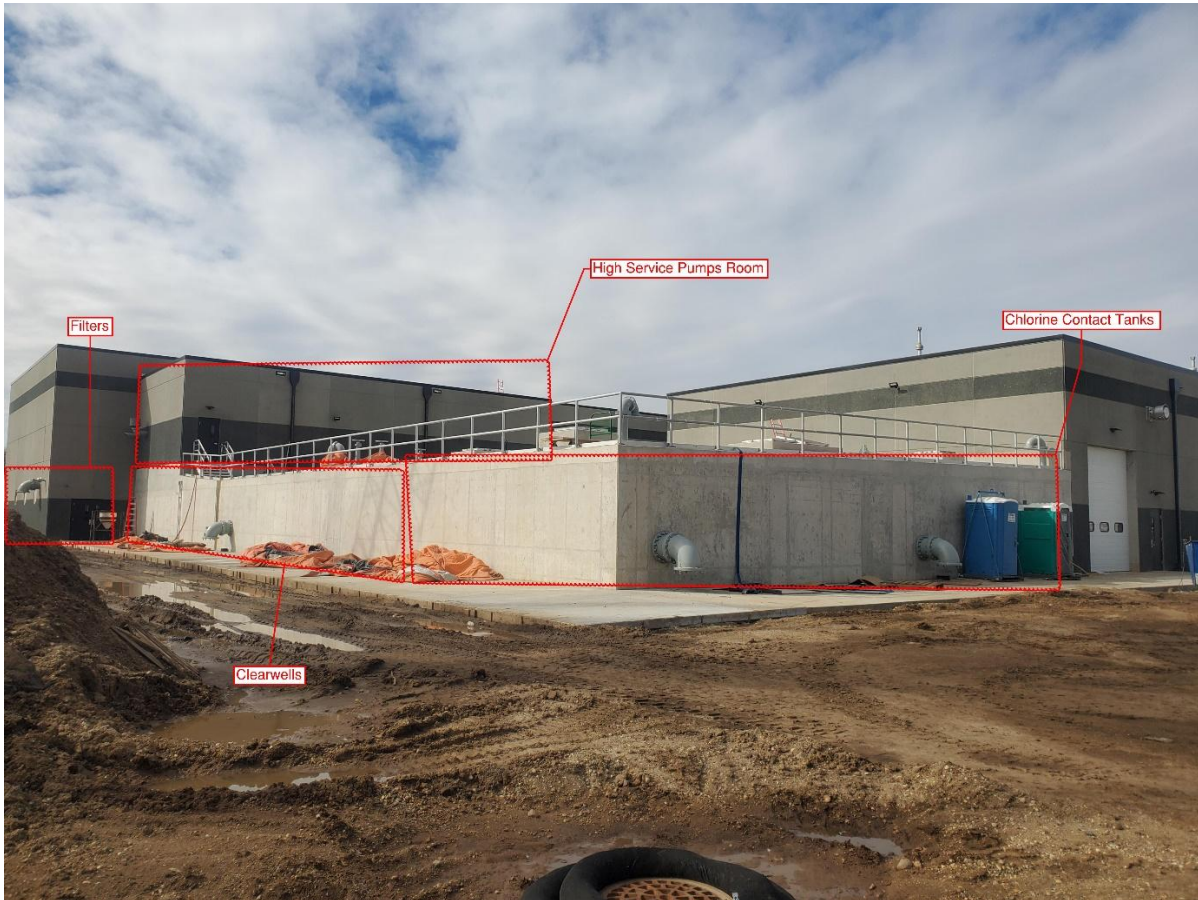
Corner view of a newly-constructed surface water treatment plant, with major features highlighted.
