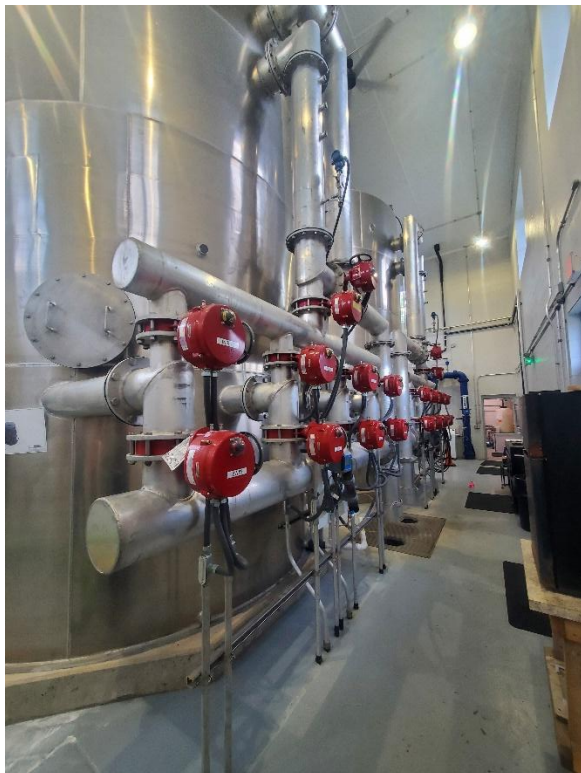
Filter units of a new groundwater treatment plant.
