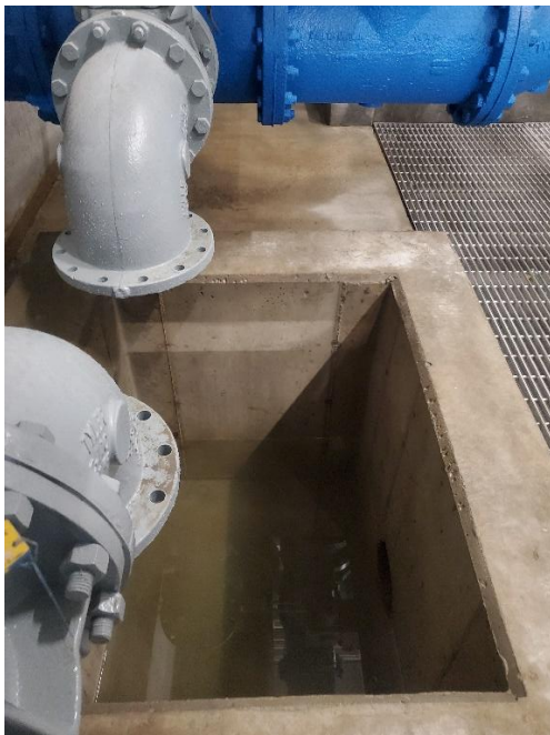
Wastewater collection in the filter pipe gallery of a new surface water treatment plant, constructed primarily in 2025 using DWSRF funds. Filter effluent diversion to waste is shown on the left and backwash water collection is shown on the right.
