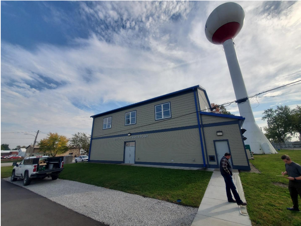
New groundwater treatment plant, constructed primarily in 2024 and 2025 using DWSRF funds.
