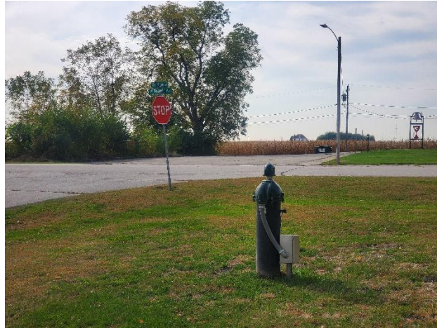
Buried sand and gravel public water supply well, drilled to a depth of approximately 265 feet below the existing round surface.
