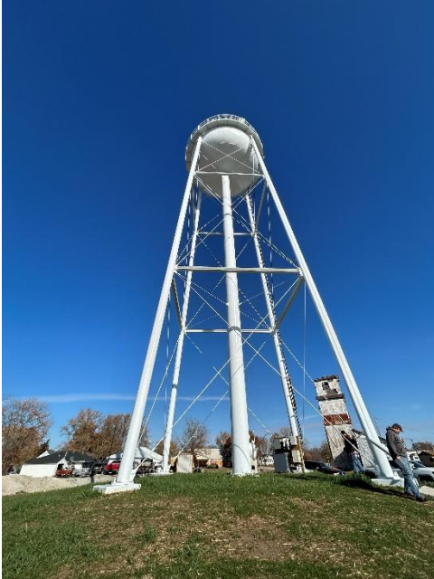
New 75,000-gallon elevated storage tank with water main for distribution system incorporation, constructed primarily in 2025 using DWSRF funds. The existing 50,000-gallon elevated storage tank was demolished due to age and safety conditions.
