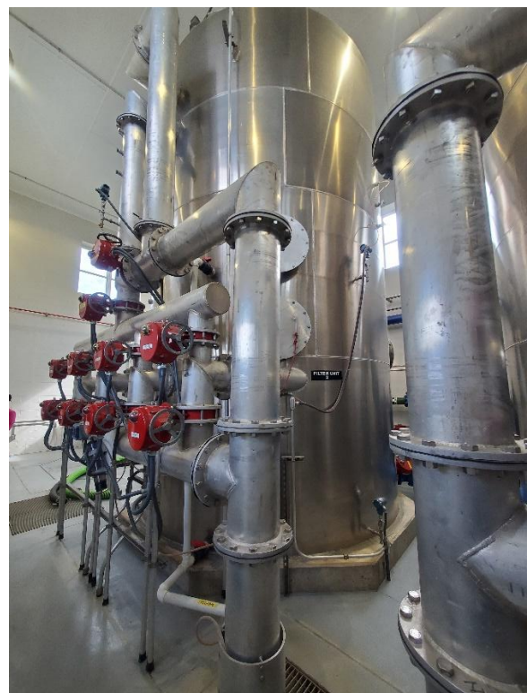
Filter units of a new groundwater treatment plant.
