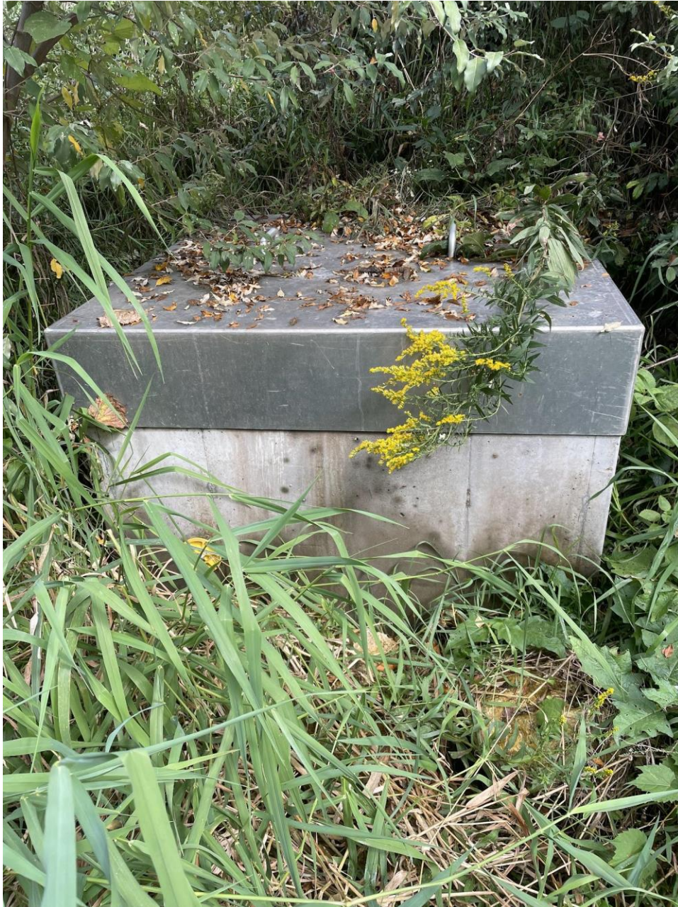
Figure 5. Site 3. Outfall upstream.
