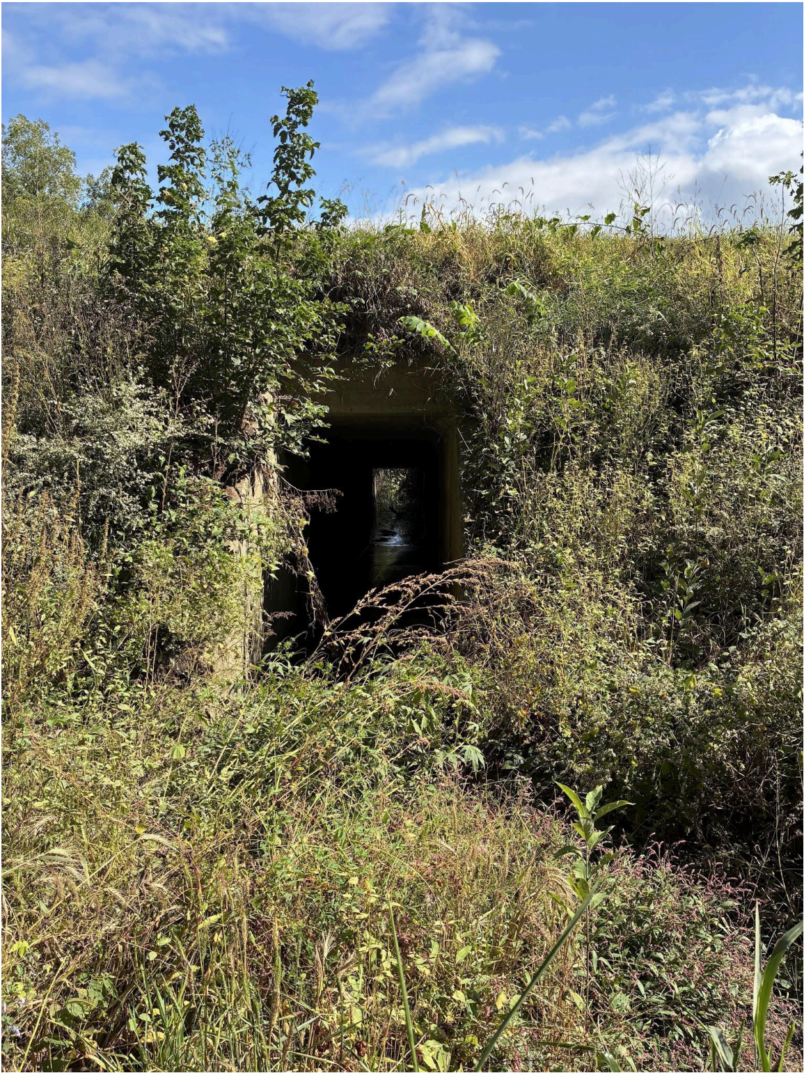
Figure 4. Site #2 looking downstream.
