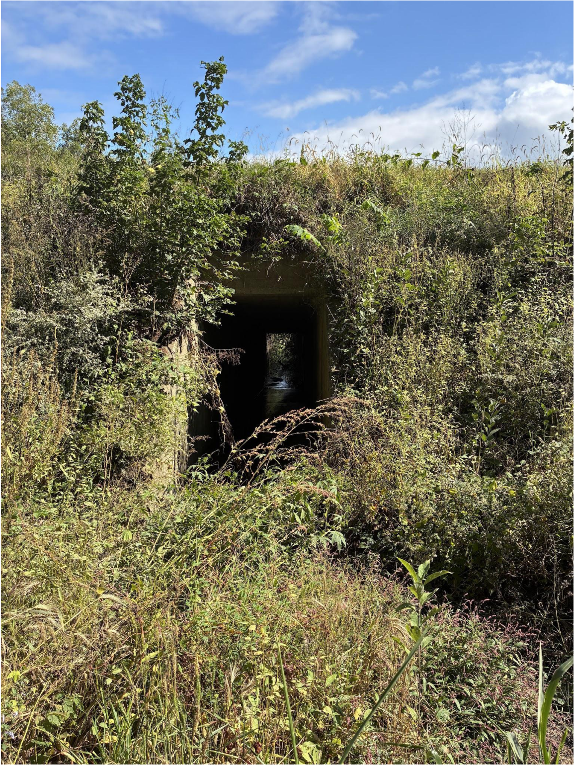
Figure 4. Site #2 looking downstream.
