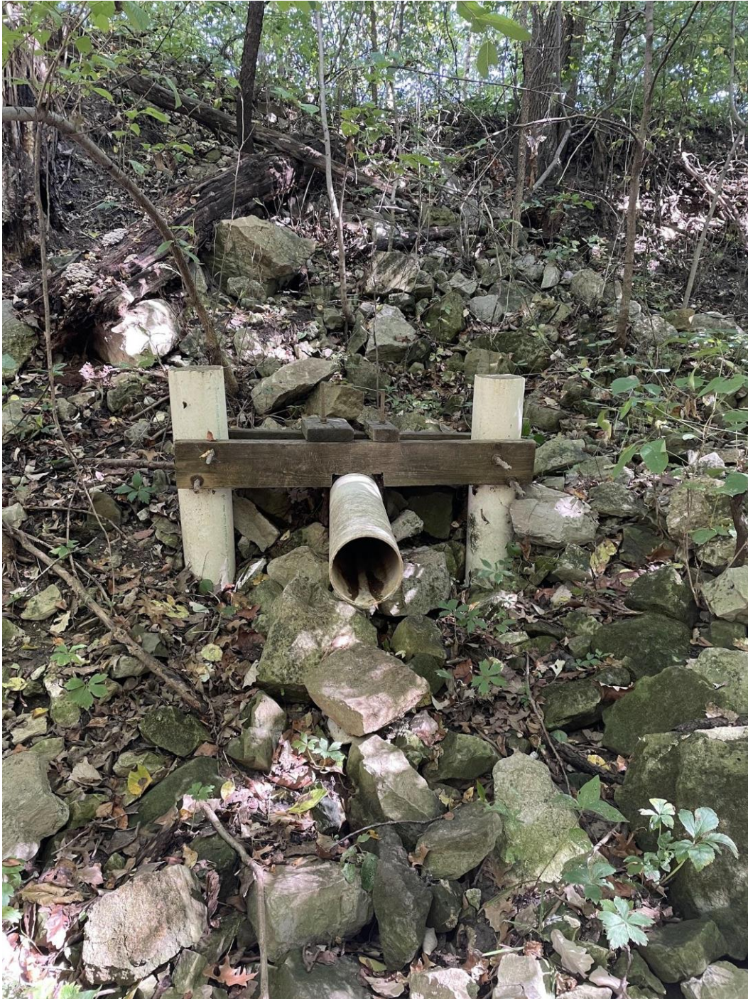
Figure 1. Site #1. Facility's outfall into Unnamed Tributary.
