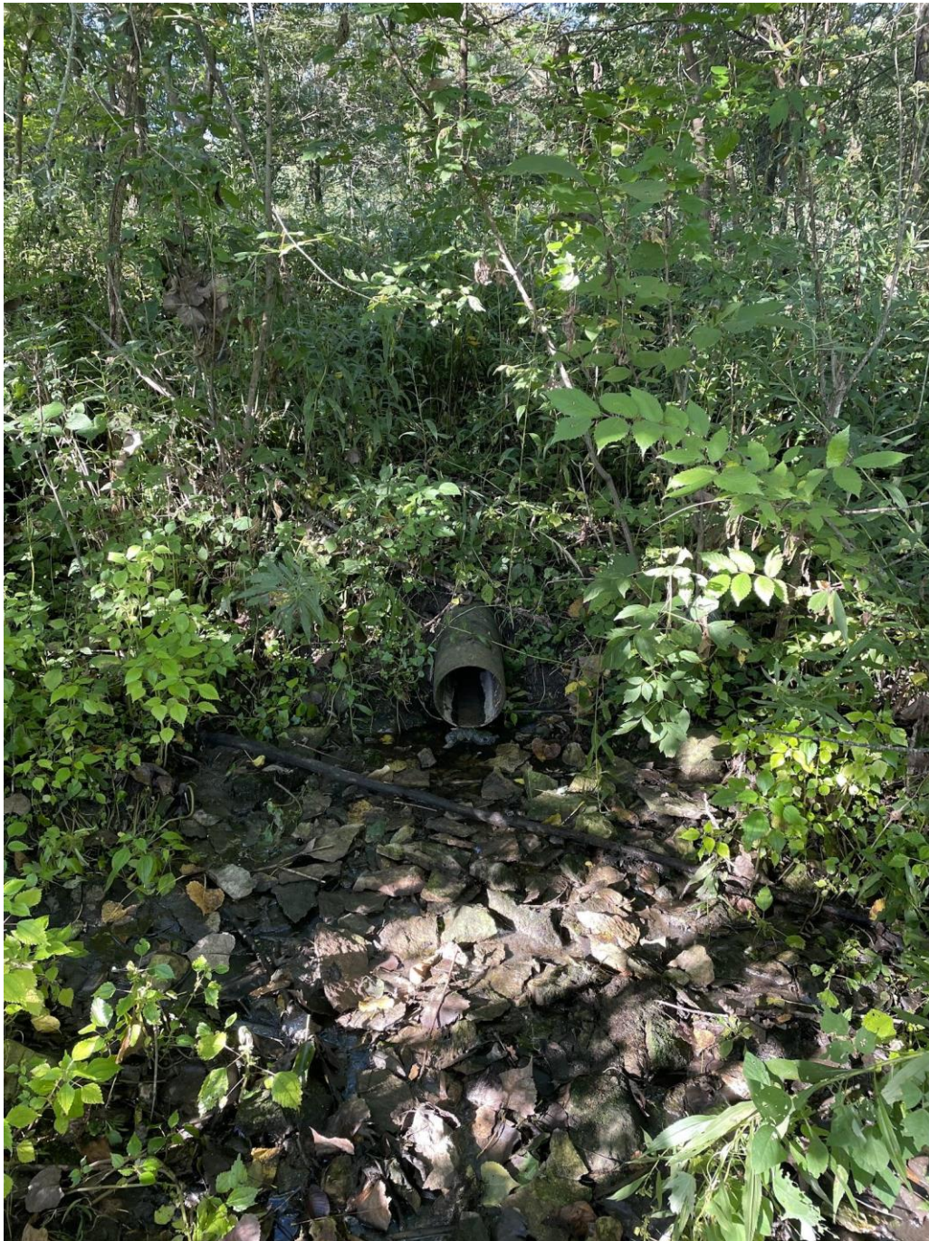
Figure 2. Site #2 looking upstream at the outfall.
