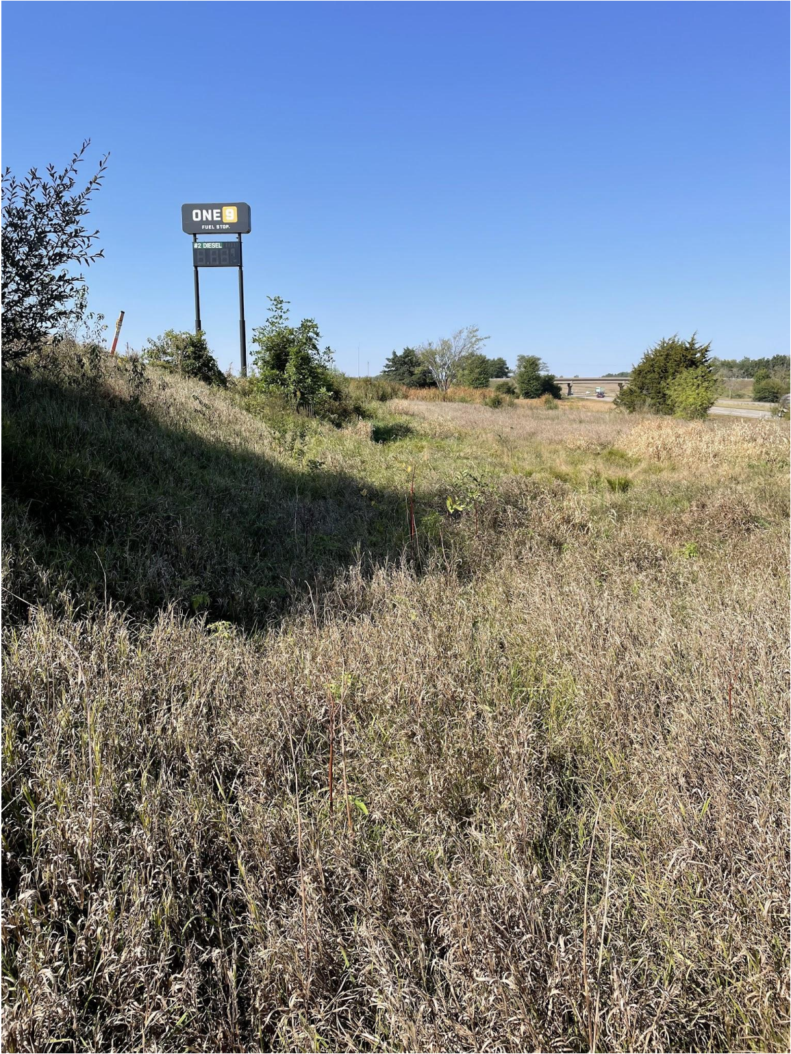
Figure 2. Outfall looking upstream from the outfall.
