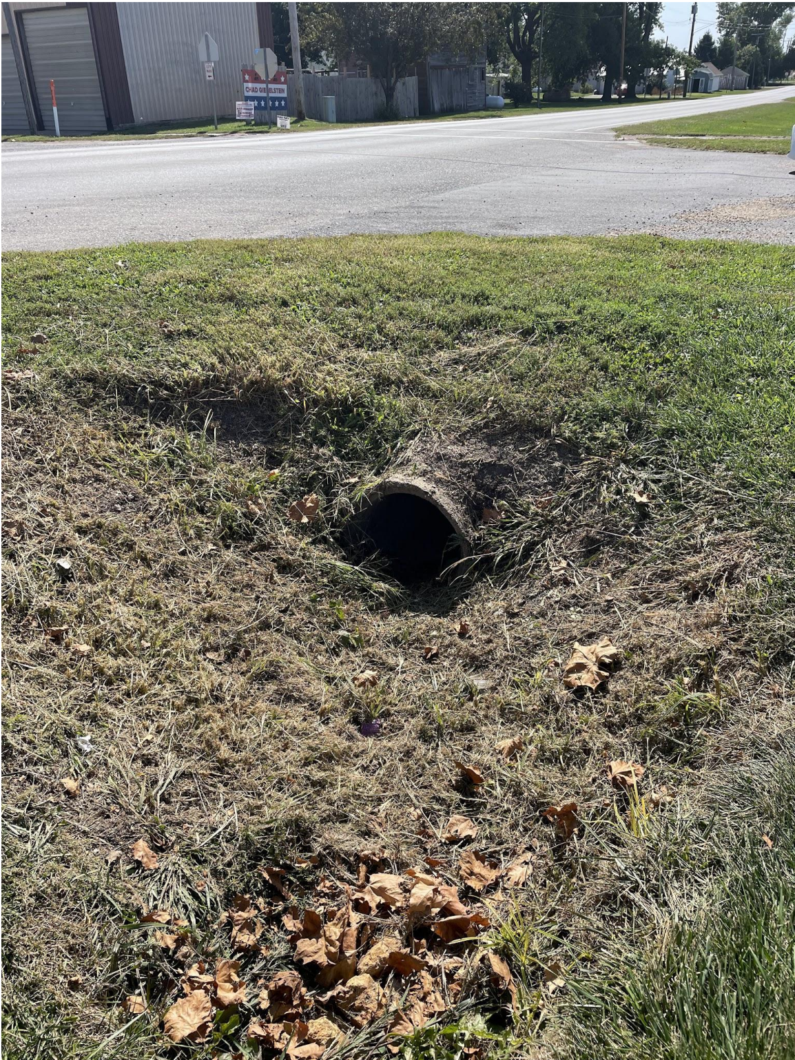
Figure 2. Site #1 looking downstream.
