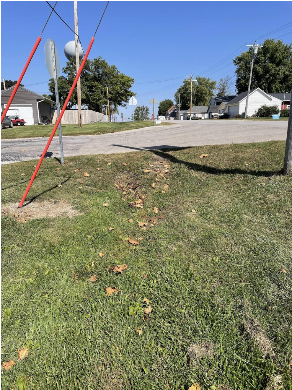
Figure 3. Site #2 Looking upstream at the outfall.
