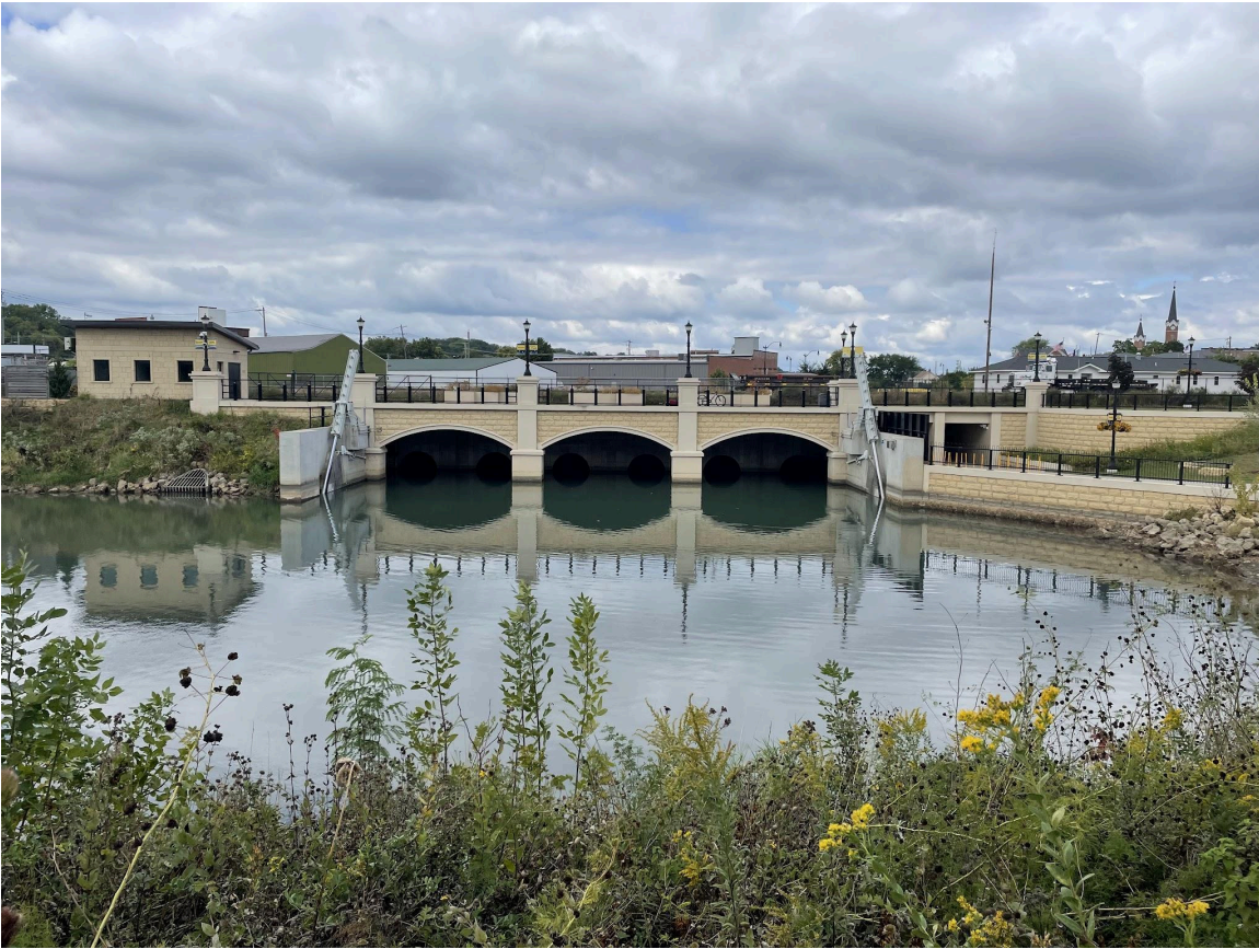
Figure 3. Site #2 looking upstream at the flood control structure.
