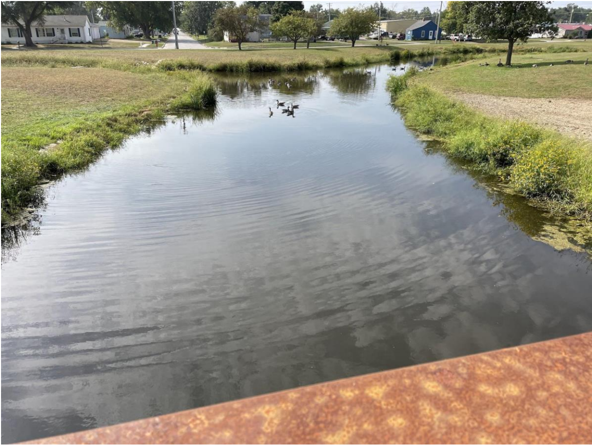
Figure 2. Site #2 looking upstream from a bridge.
