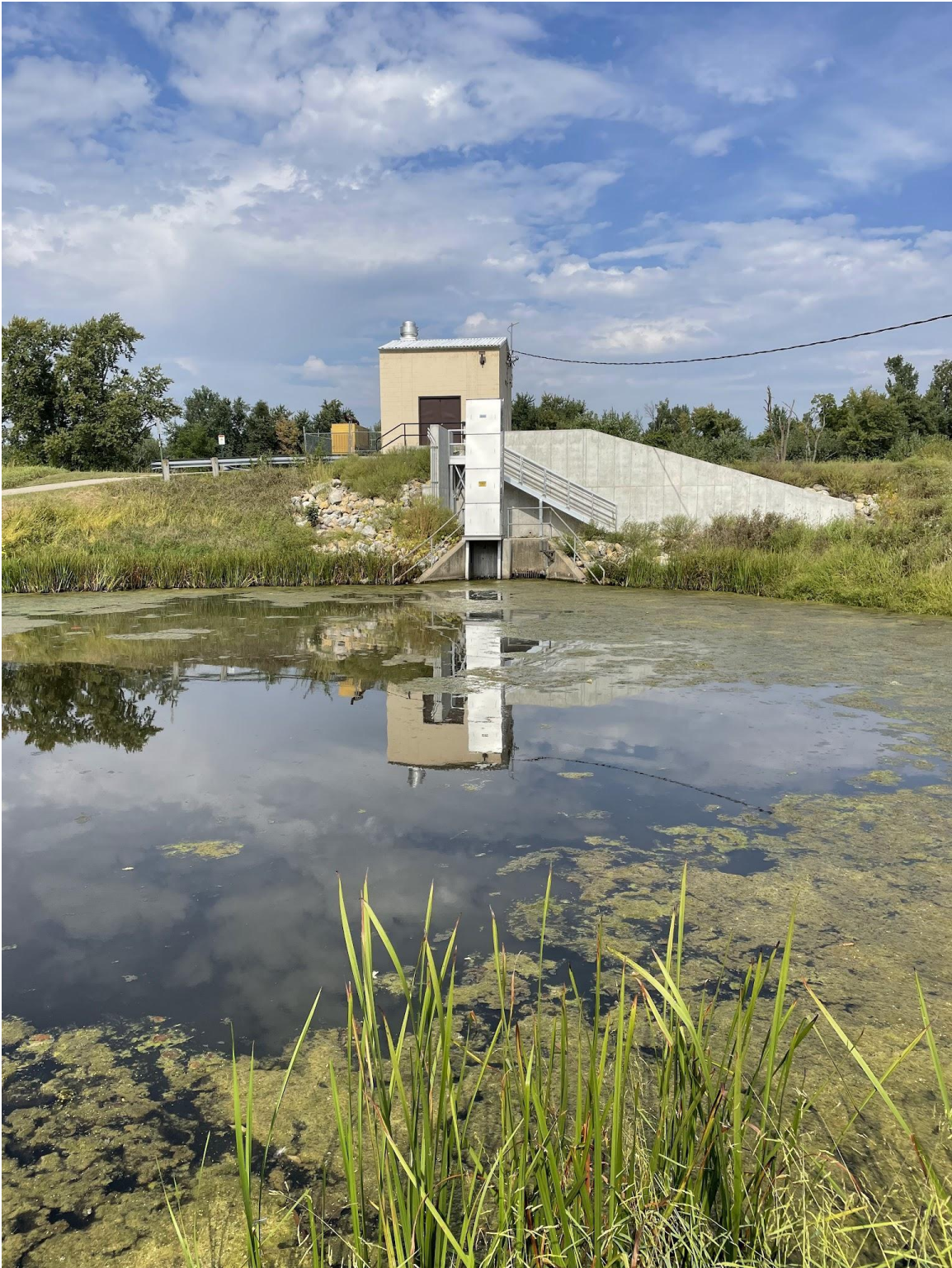
Figure 1. Site #1 looking downstream at the flood control structure.
