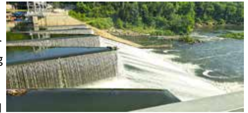
View of Delhi Dam spillway from the overlook
