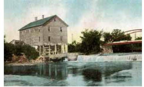
Hopkinton Mill was first a sawmill, then a flour mill, and finally a generator plant for electricity.
