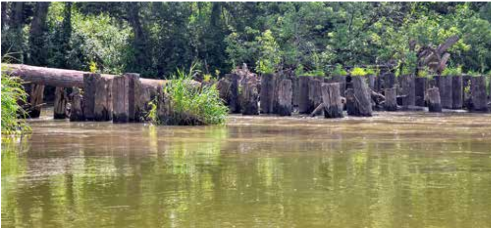
Posts blocking inlet from Plum Creek river-left
