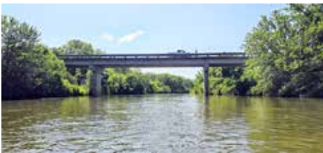
Quarter Road Bridge upstream of Pioneer Road Access
