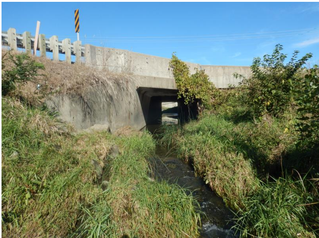
Figure 4. 319-4 Upstream looking upstream.
