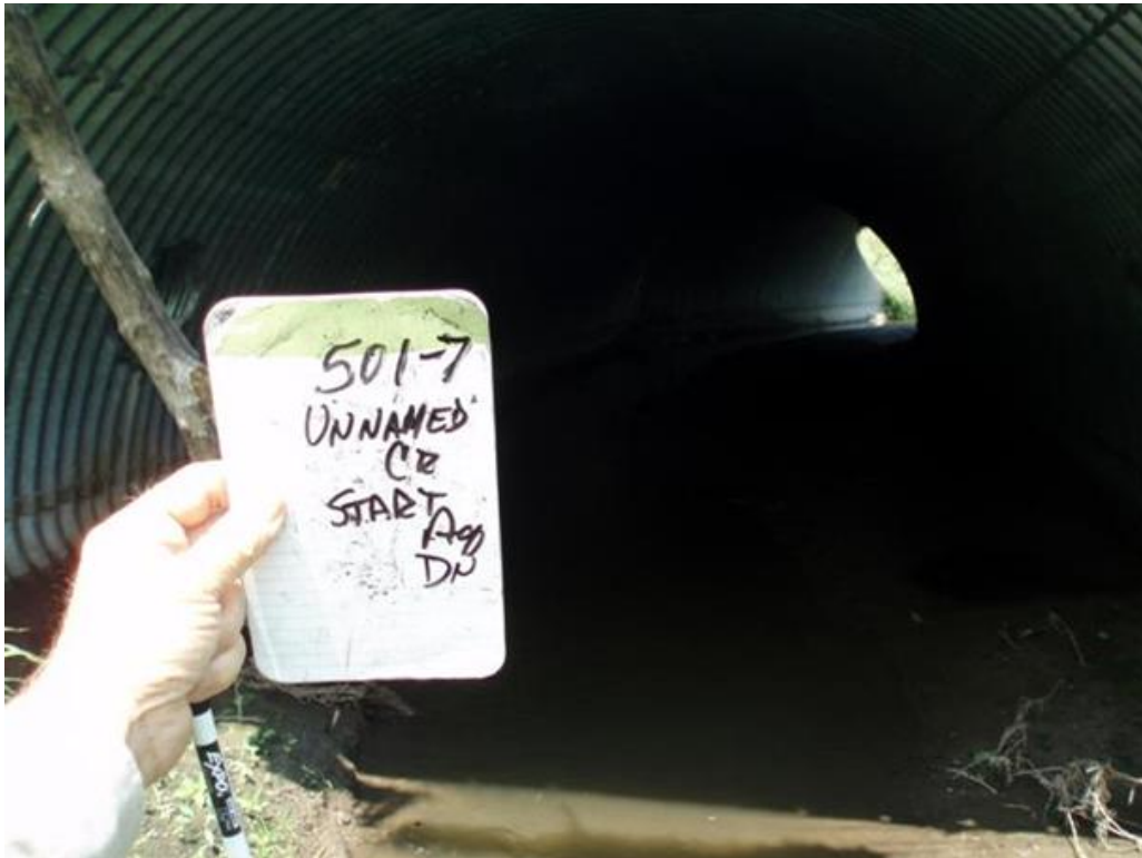
Figure 3. 501-7 Start of aquatic assessment looking downstream.
