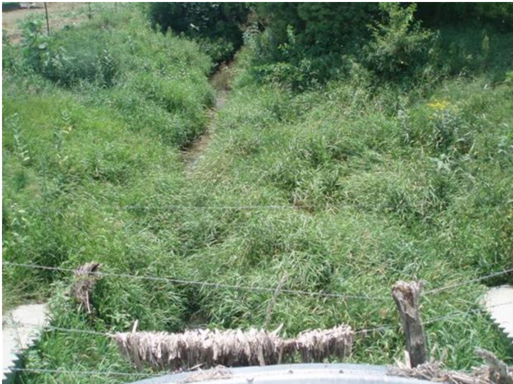
Figure 2. 501-7 Road looking upstream #2.
