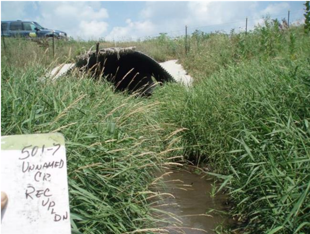
Figure 14. 501-7 Upstream recreation site looking downstream.
