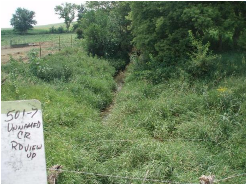
Figure 1. 501-7 Road looking upstream.
