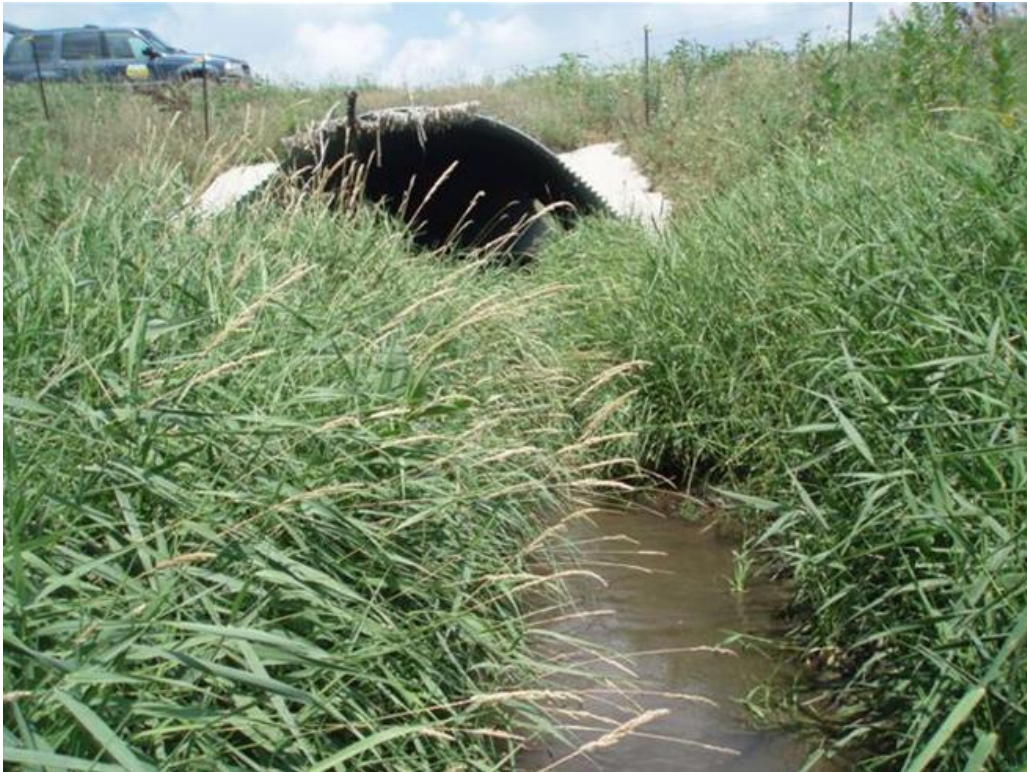
Figure 15. 501-7 Upstream recreation site looking downstream #2.
