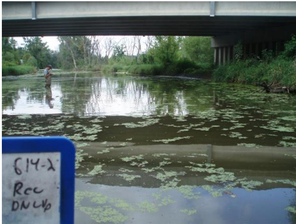
Figure 24. 614-2 Downstream recreation site looking upstream.
