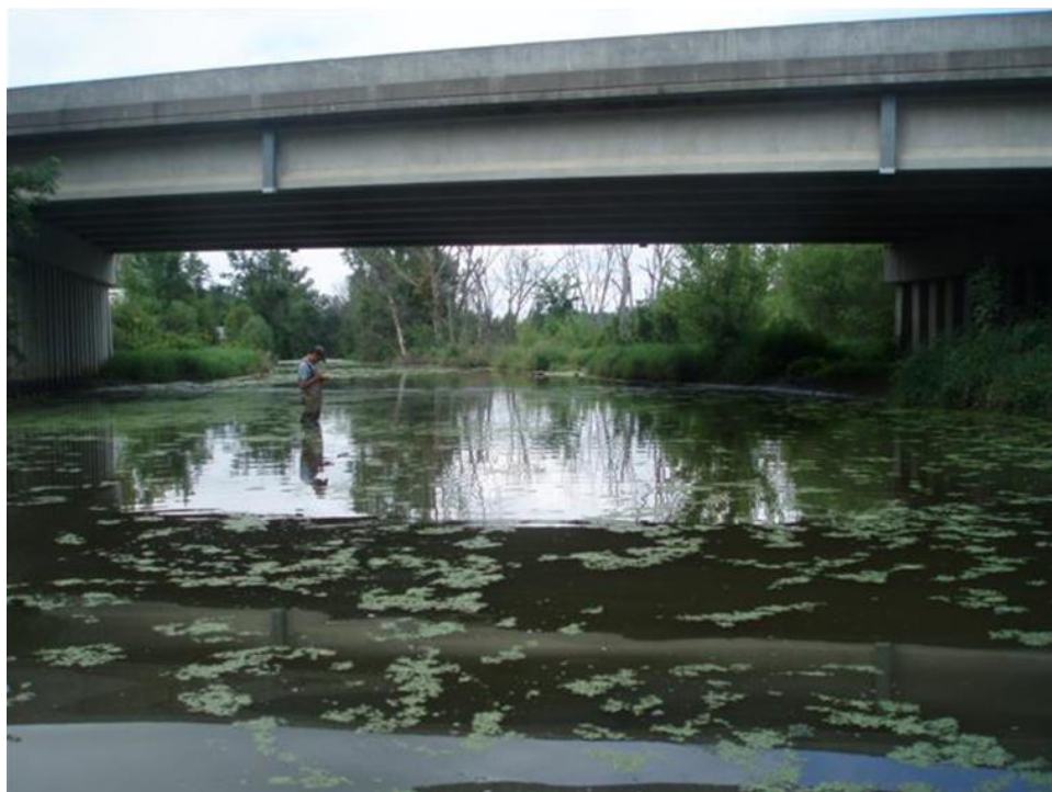
Figure 25. 614-2 Downstream recreation site looking upstream #2.
