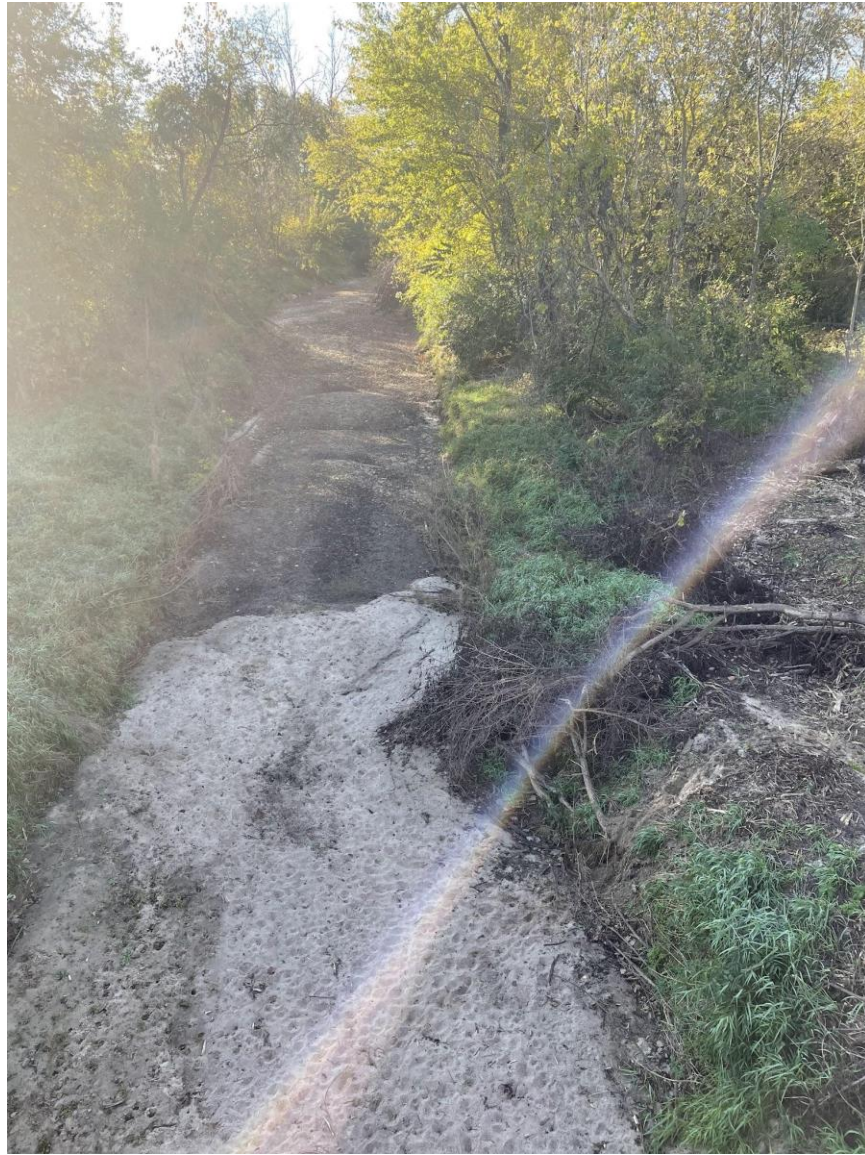
Figure 16. 614-2 Bridge looking downstream, supplemental visit.
