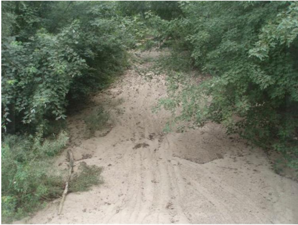
Figure 4. 614-1 Bridge looking downstream.
