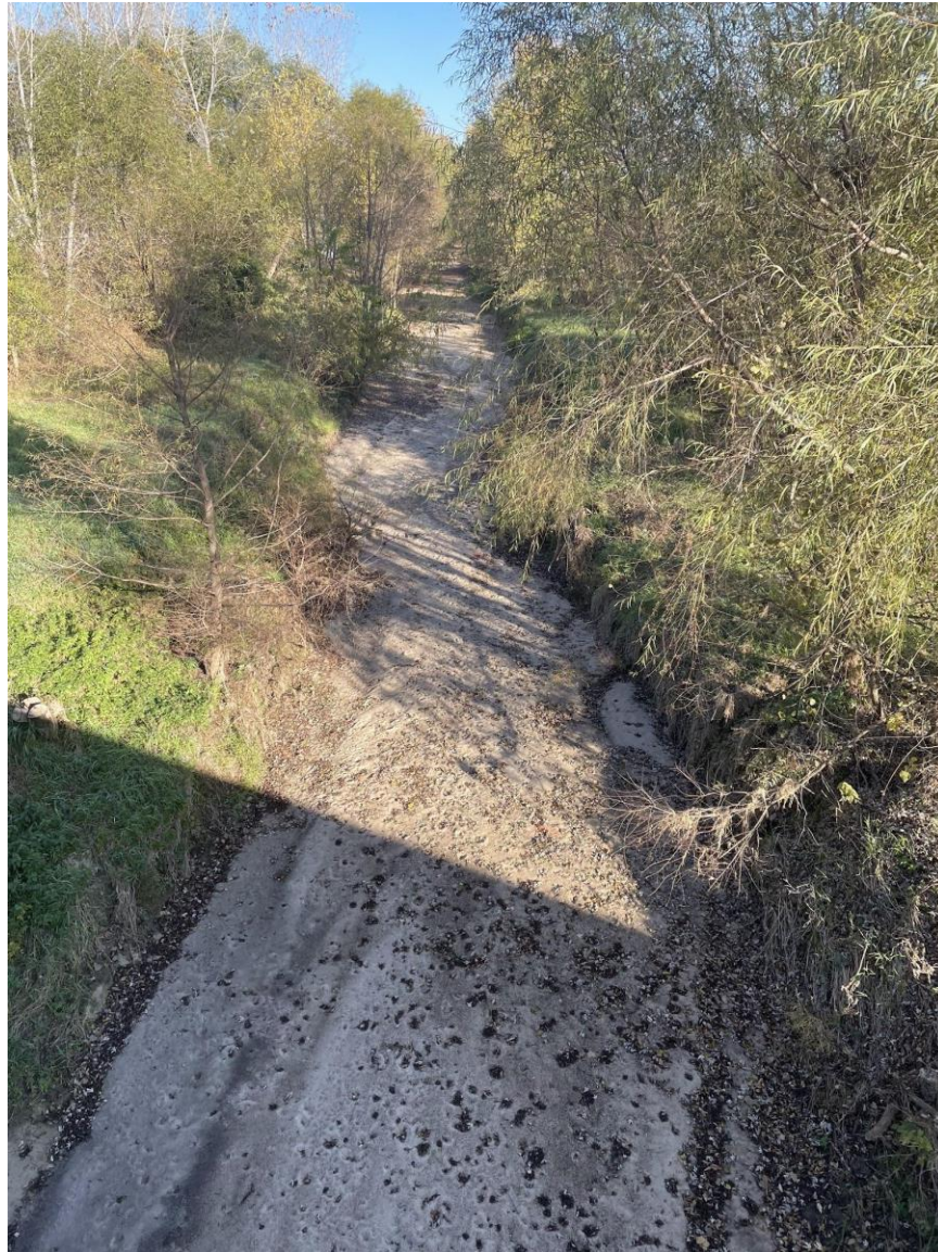
Figure 13. 614-2 Bridge looking upstream, supplemental visit.
