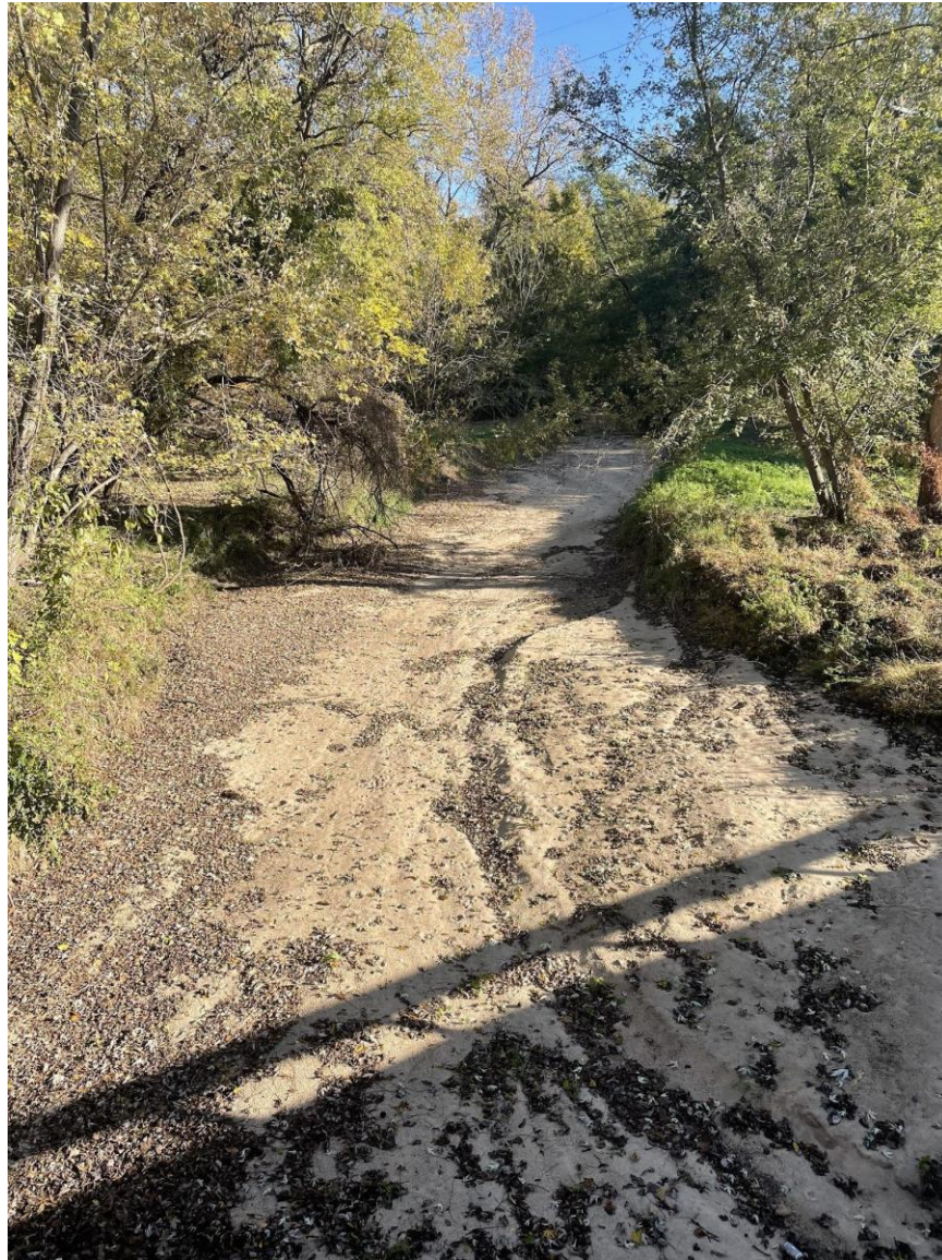
Figure 5. 614-1 Bridge looking downstream, supplemental visit.
