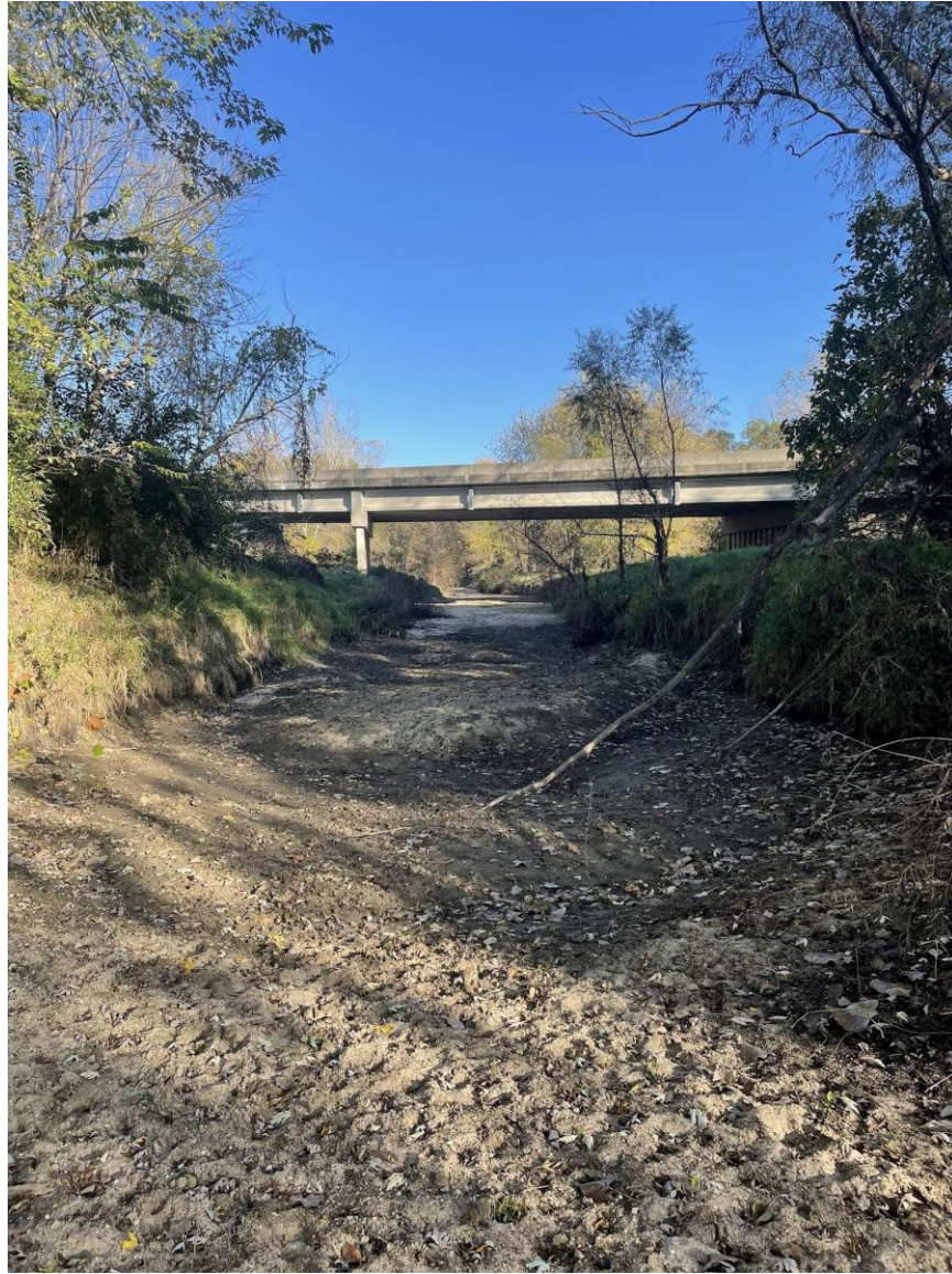
Figure 26. 614-2 Downstream recreation site looking upstream, supplemental visit.
