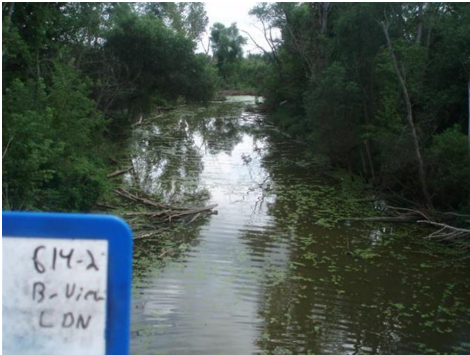
Figure 15. 614-2 Bridge looking downstream.
