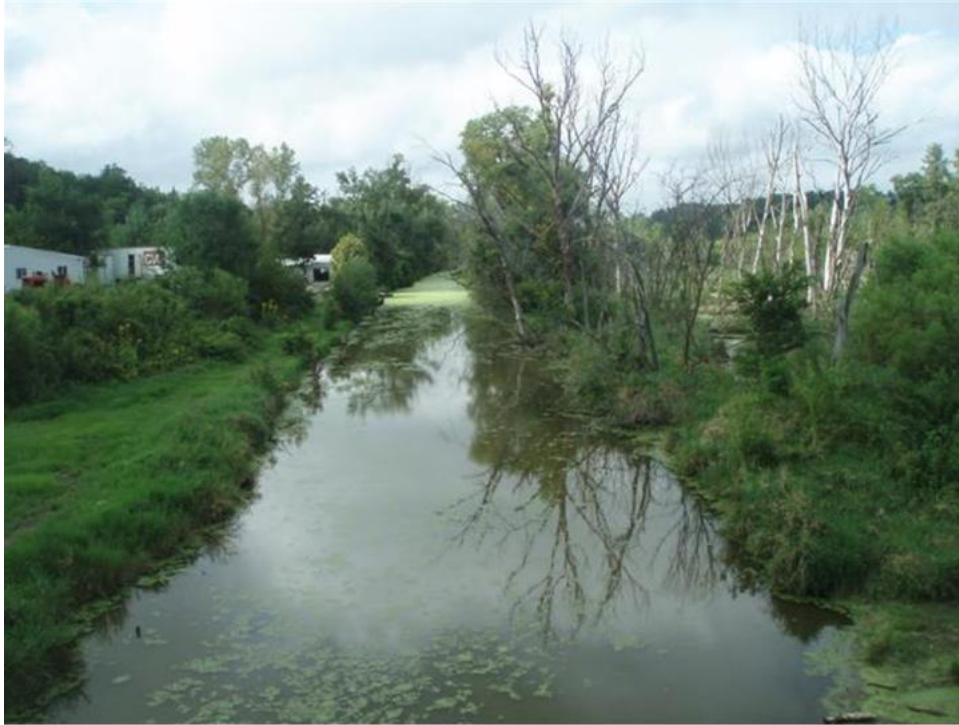
Figure 14. 614-2 Bridge looking upstream #2.
