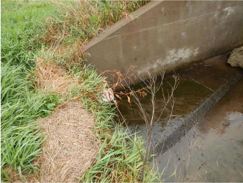
Figure 15. 1131-2 Tile line draining into culvert upstream view 2.
