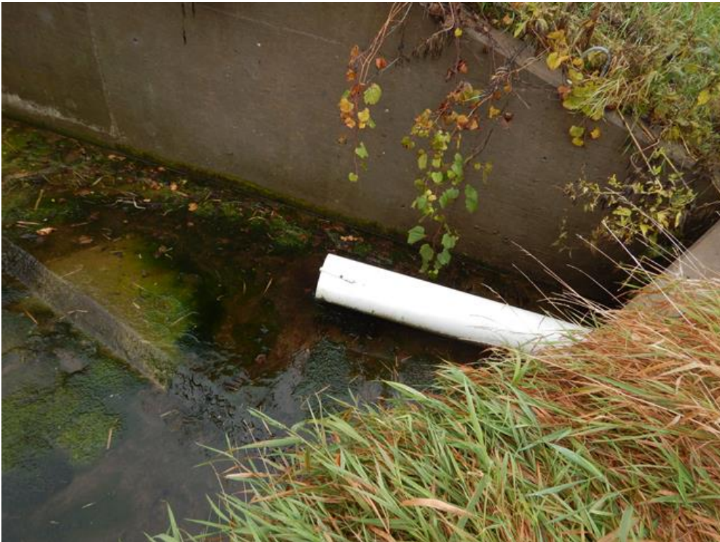
Figure 14. 1131-2 Tile line draining into culvert upstream.
