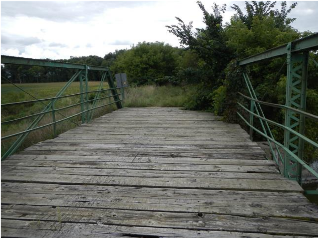
Figure 11. 1055-4 Bridge at Swan Lake outlet.
