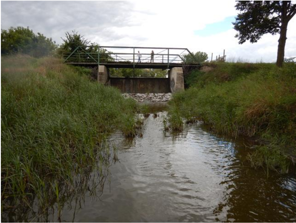
Figure 9. 1055-4 Recreational use assessment downstream looking upstream.
