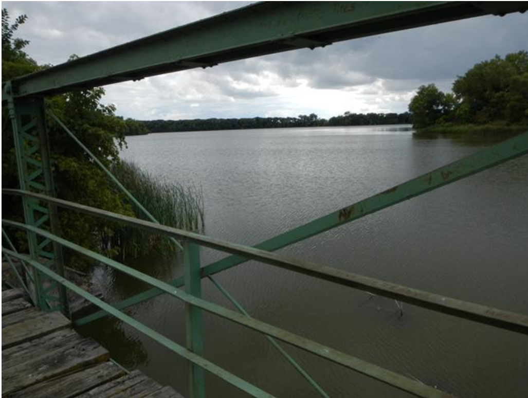
Figure 13. 1055-4 Looking at Swan Lake from the bridge.
