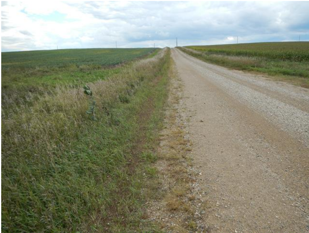
Figure 21. 1055-5 Road facing east.
