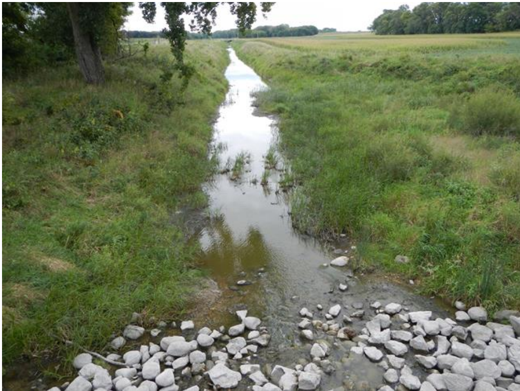
Figure 8. 1055-4 Recreational use assessment midpoint looking downstream view 2.
