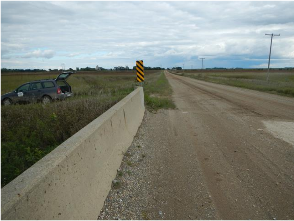
Figure 35. 1055-7 Road facing east.
