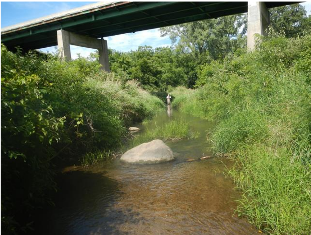
Figure 10. 1156-3 Recreational use assessment upstream looking downstream.
