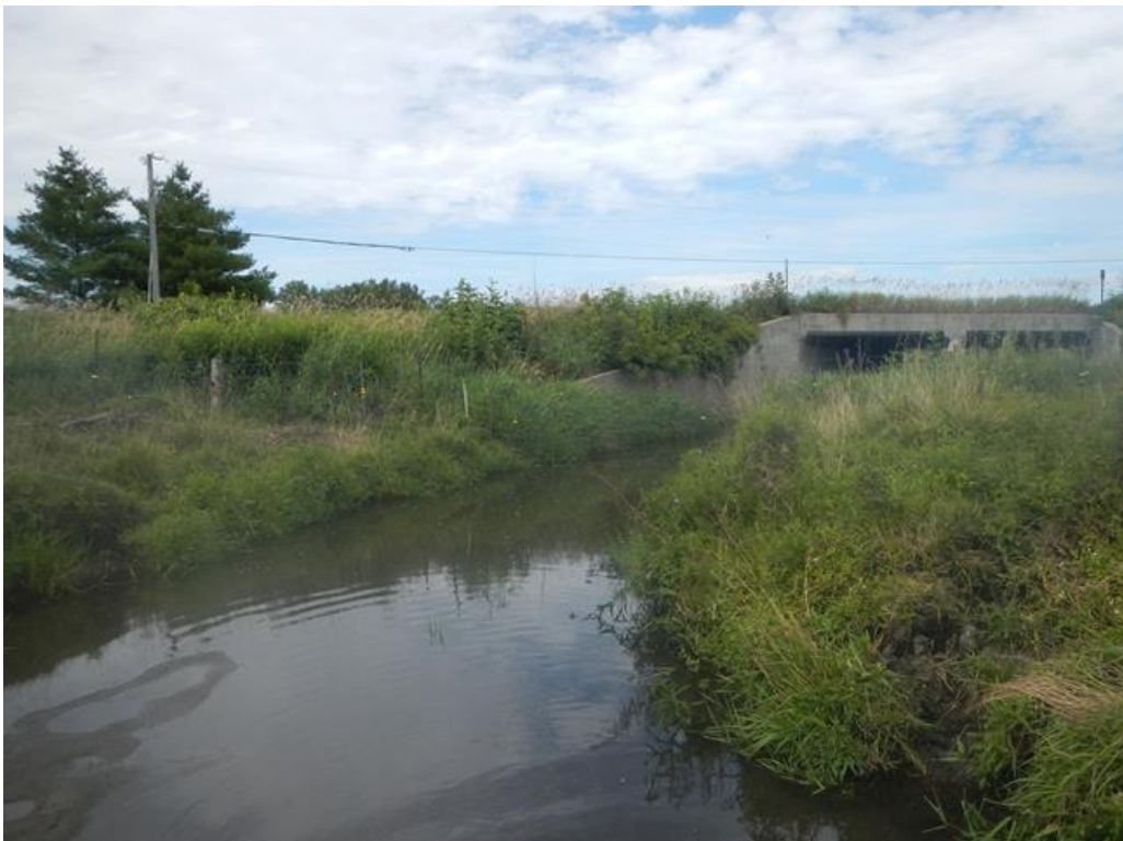
Figure 2. 1156-2 Recreational use assessment upstream looking downstream.
