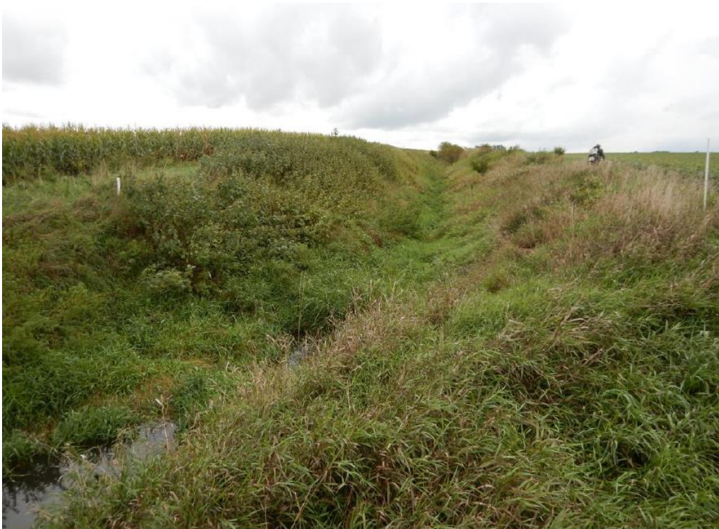
Figure 4. 1055-1 Bank view looking downstream.
