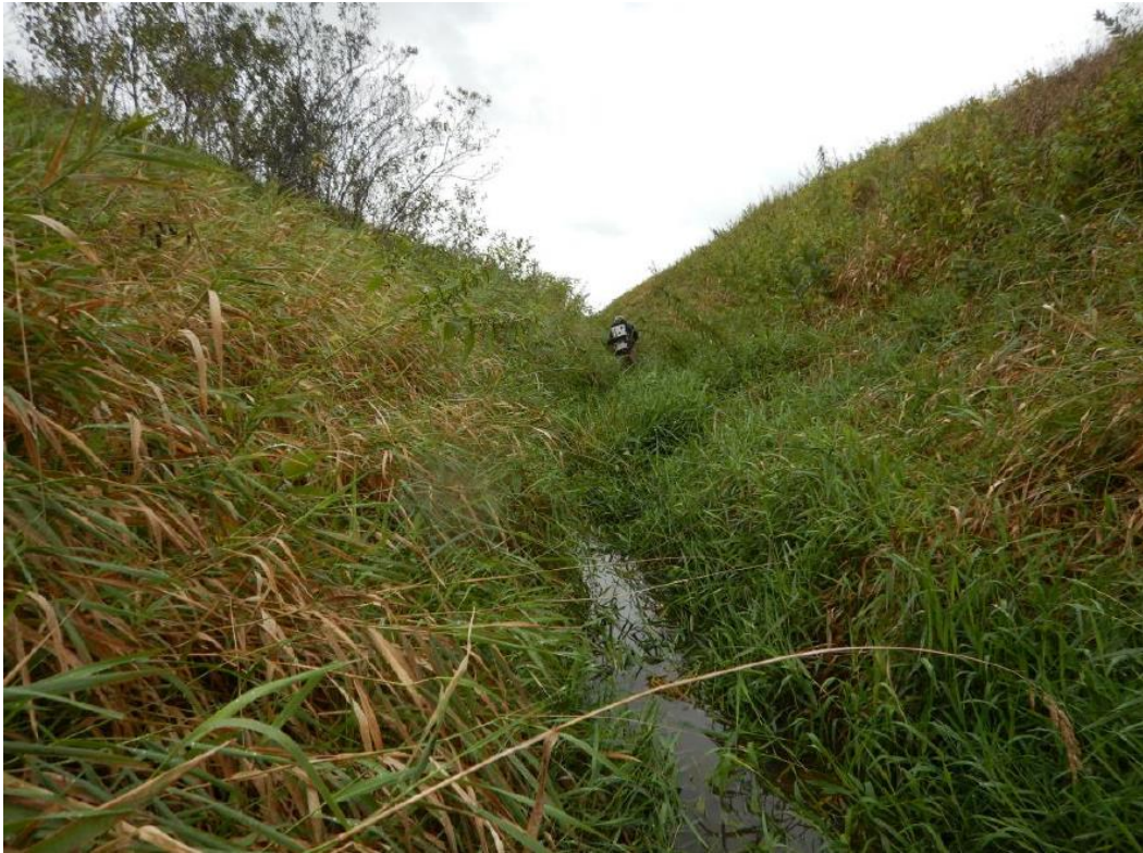
Figure 7. 1055-1 Start of aquatic use assessment looking upstream.
