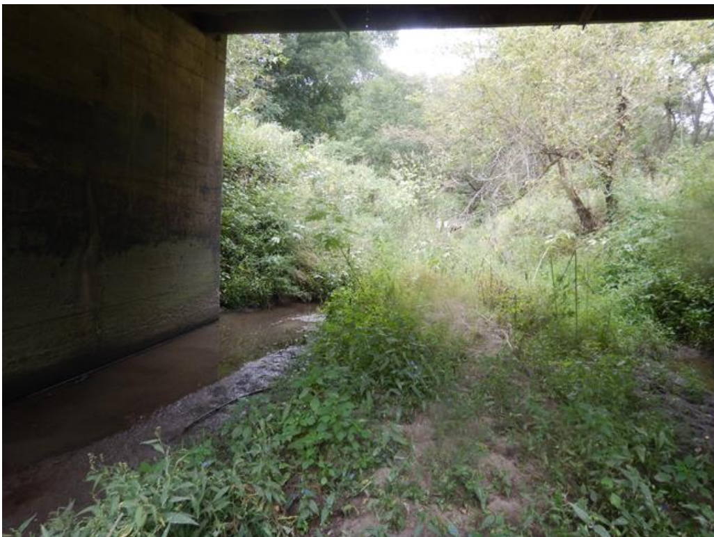
Figure 14. 1288-2 Start of aquatic assessment looking upstream.
