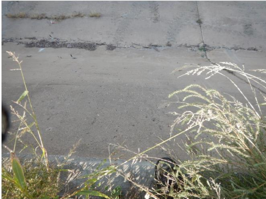
Figure 4. 1273-1 Looking down into concrete ditch.
