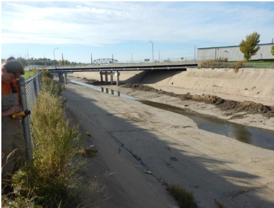
Figure 2. 1273-1 Concrete waterway looking downstream.
