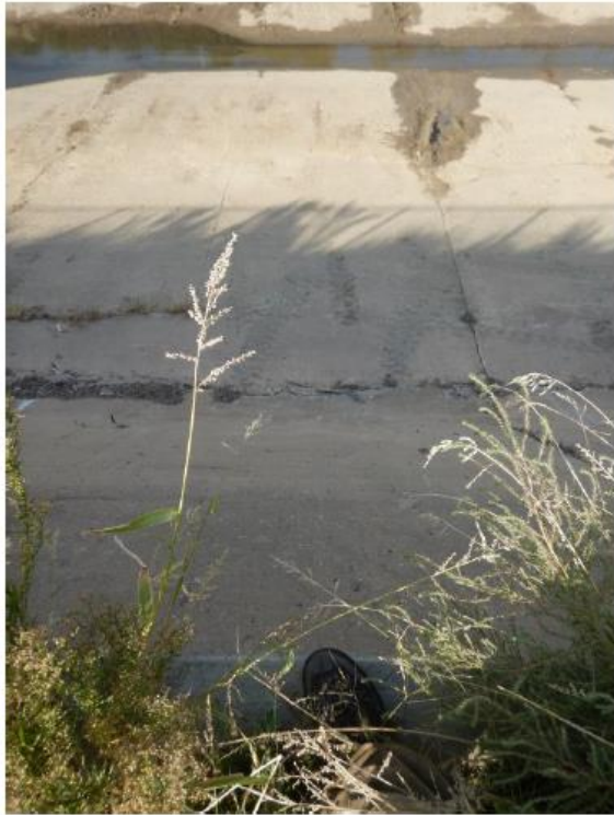
Figure 3. 1273-1 Looking down at concrete waterway.
