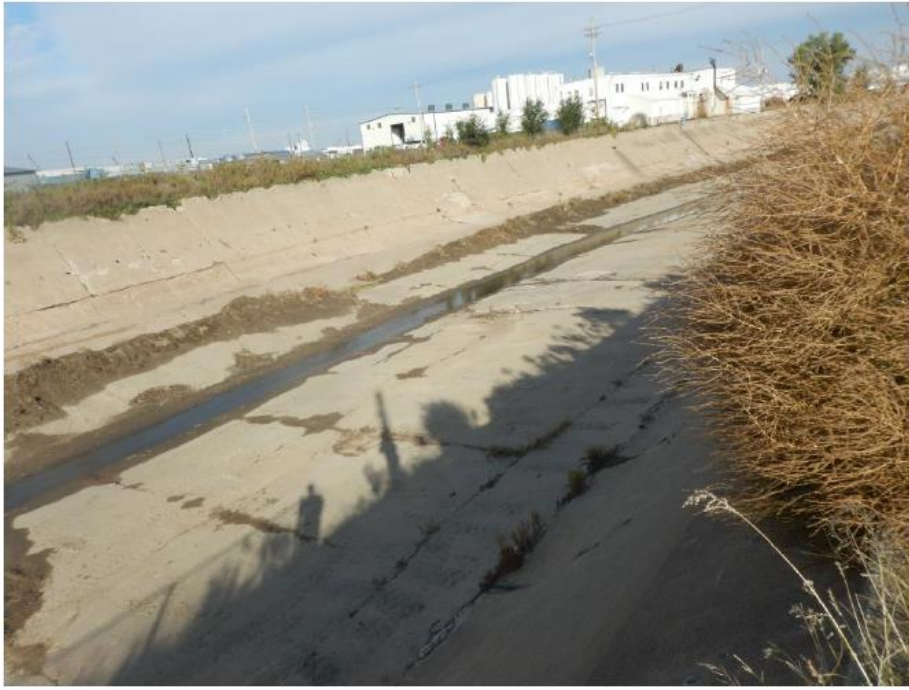
Figure 1. 1273-1 Concrete waterway looking upstream.
