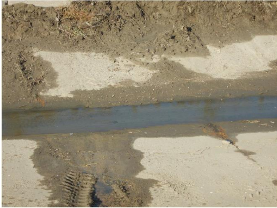
Figure 5. 1273-1 Water flowing in concrete waterway.
