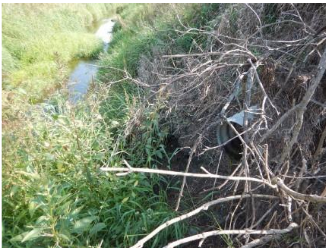
Figure 14. 1287-1 View of outfall looking upstream.
