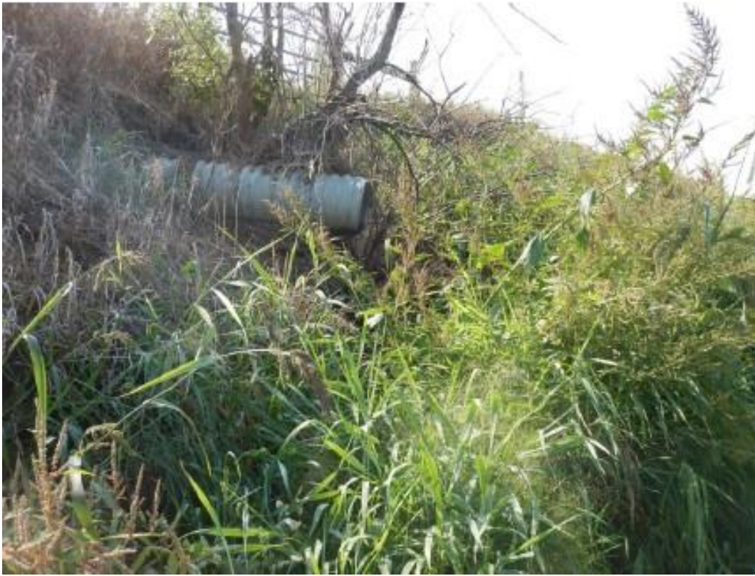
Figure 15. 1287-1 View of outfall looking downstream.
