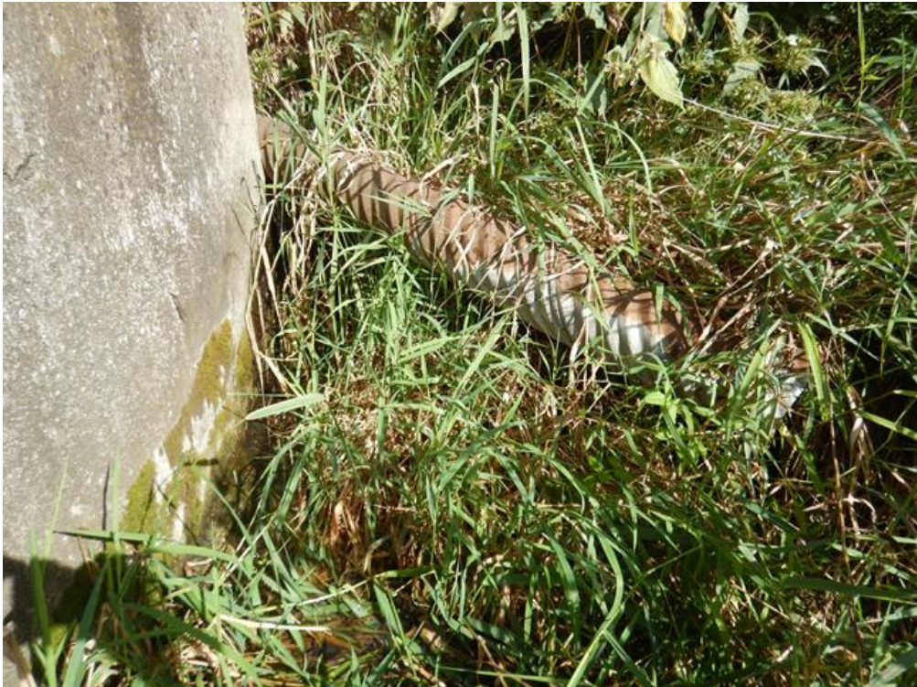
Figure 11. 1337-1 Flowing tile at north corner of drop structure.
