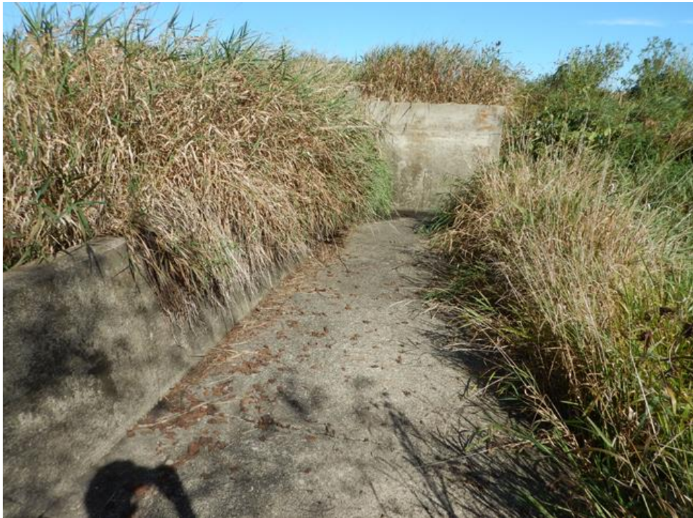
Figure 16. 1337-1 View north of drop structure.
