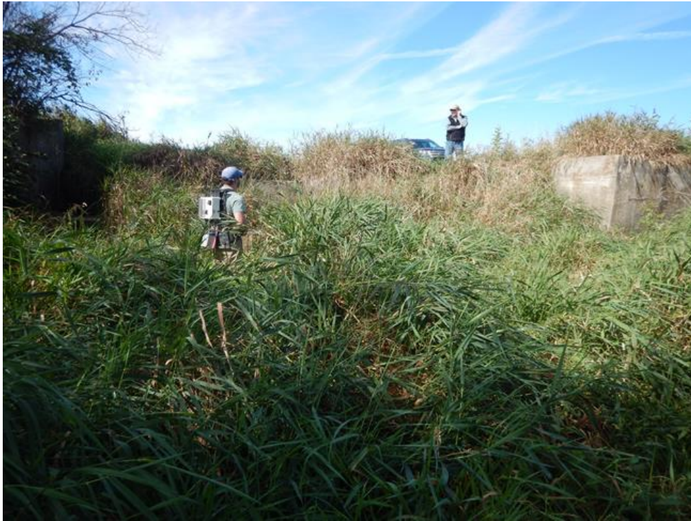
Figure 5. 1337-1 Drop structure partially visible – view west.
