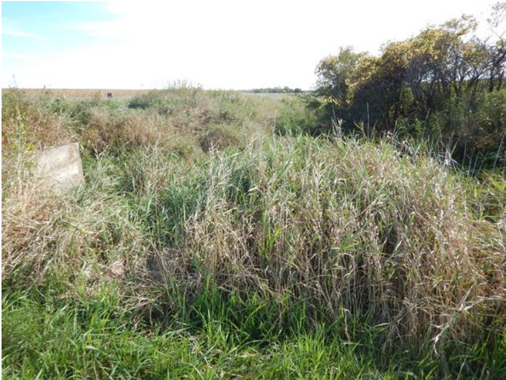
Figure 15. 1337-1 View east from edge of drop structure.
