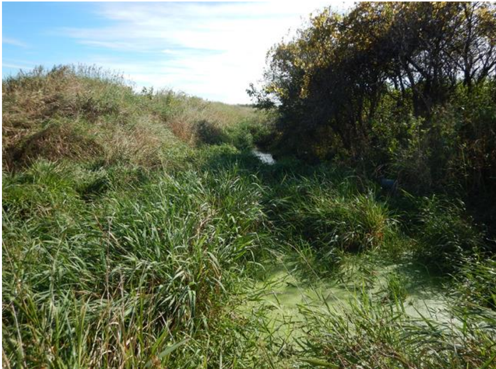
Figure 14. 1337-1 View east from drop structure.
