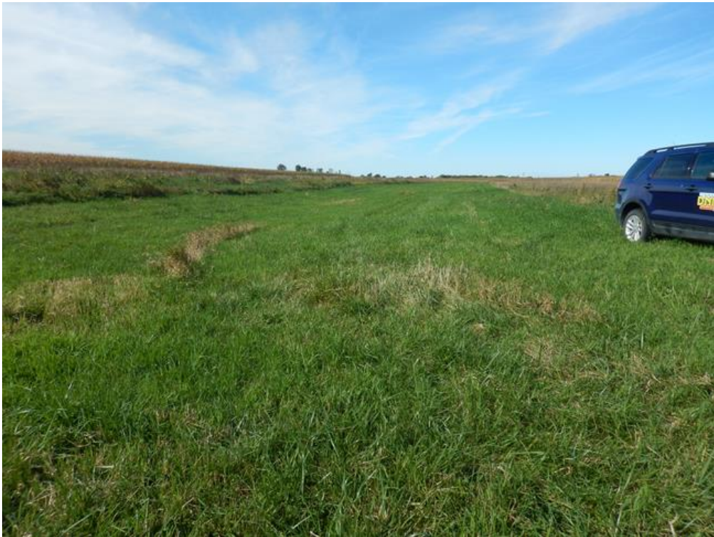
Figure 18. 1337-1 View west of grassed waterway above drop structure.
