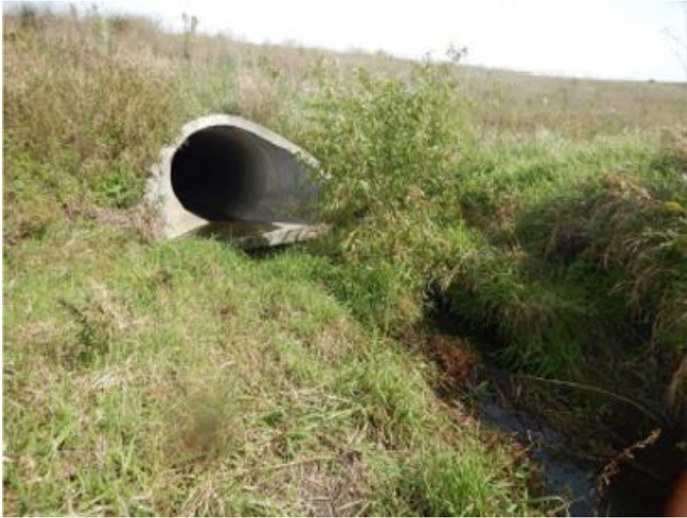
Figure 1. 1333-1 Recreational use assessment upstream looking upstream.
