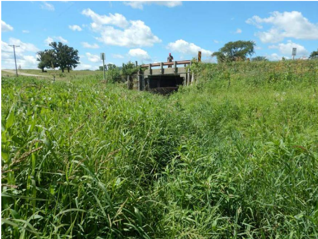
Figure 2. 1371-2 Recreational use assessment upstream looking downstream.
