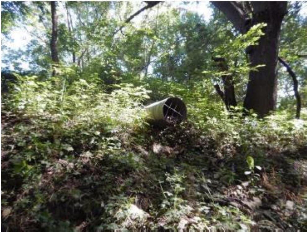
Figure 5. 1357-1 Recreational use assessment facility outfall.
