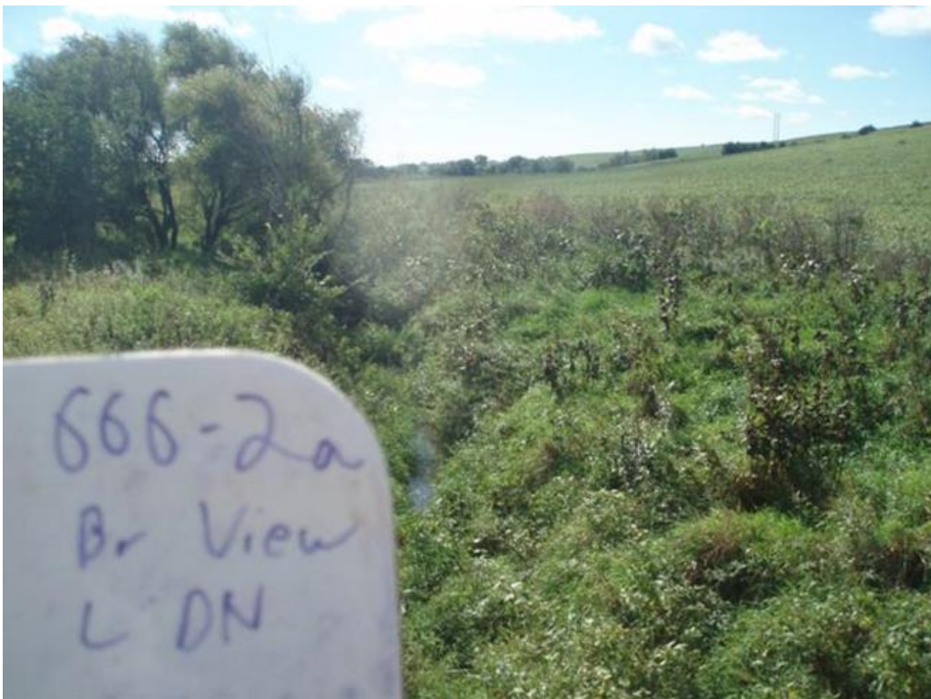
Figure 26. 666-1a Bridge view, looking downstream #2.
