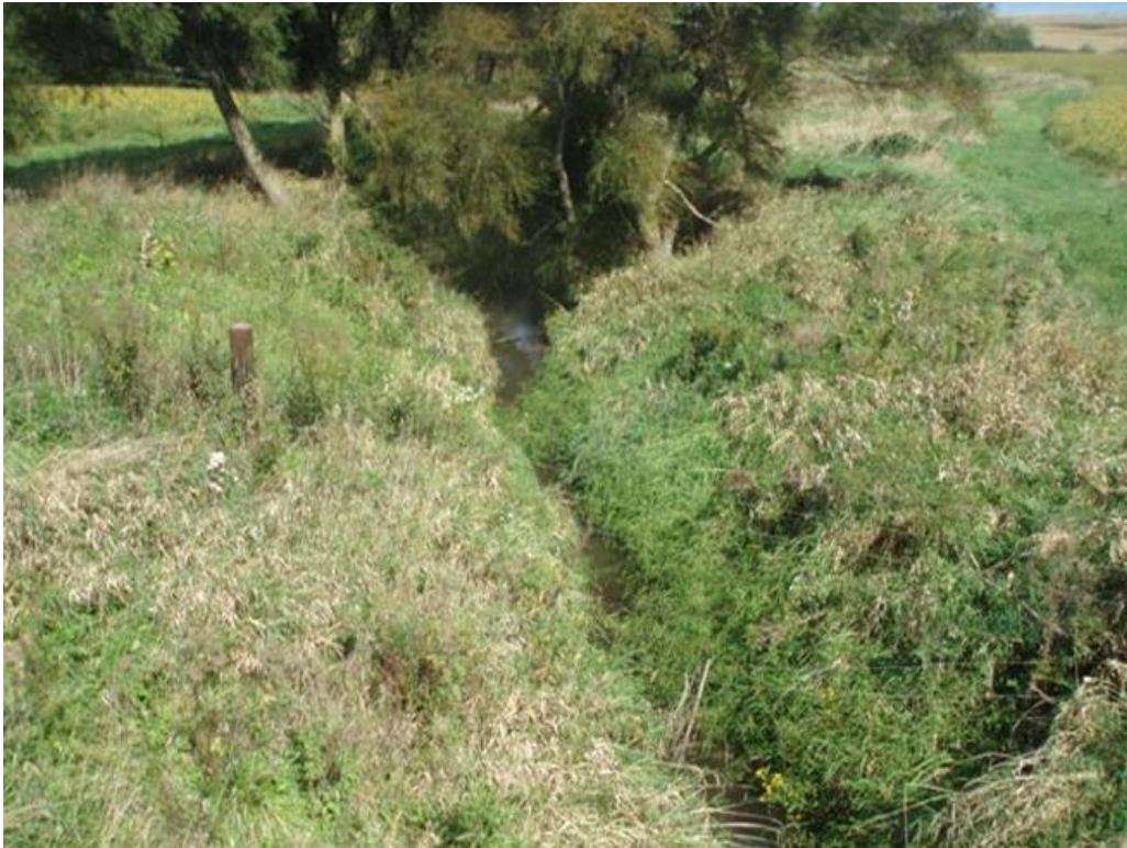
Figure 23. 666-1a Bridge view, looking upstream.
