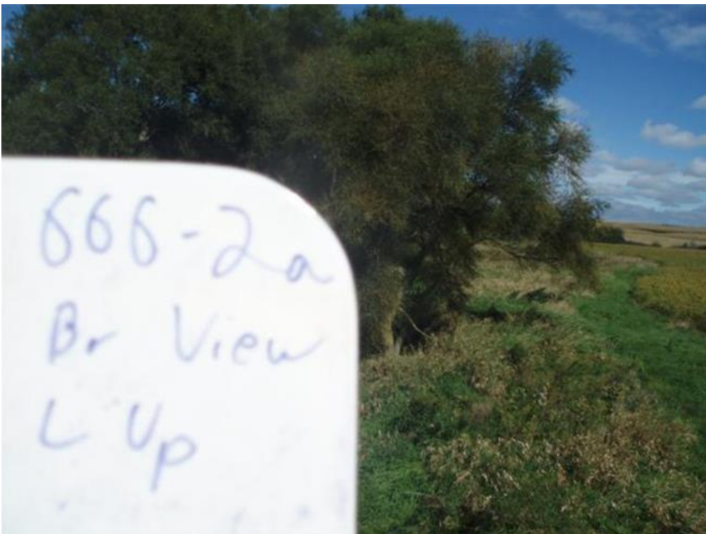
Figure 24. 666-1a Bridge view, looking upstream #2.
