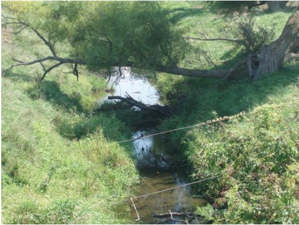
Figure 3. 666-1 Bridge view, looking downstream.
