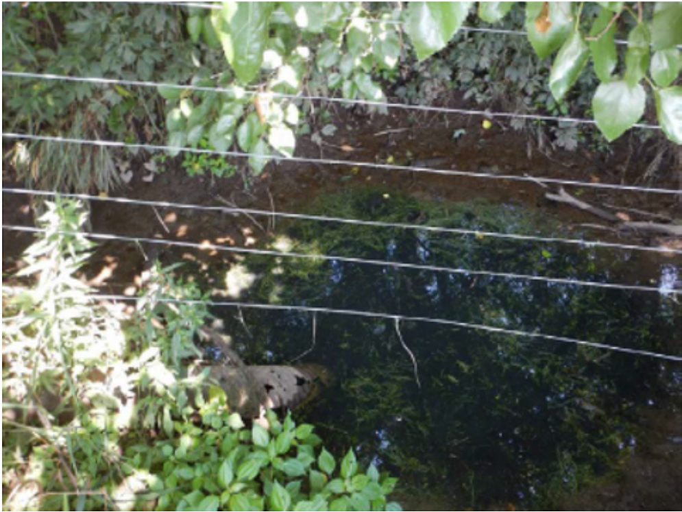
Figure 3. 1387-1 Recreational use assessment puddle under outfall.
