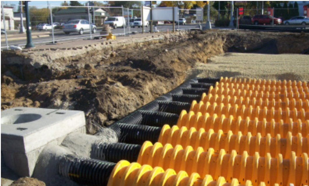
An underground detention chamber system under construction in Davenport.
