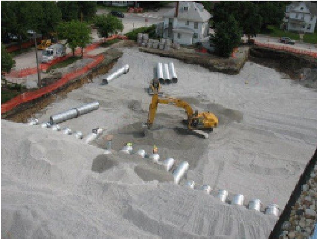
An underground detention chamber system under construction in Davenport.
