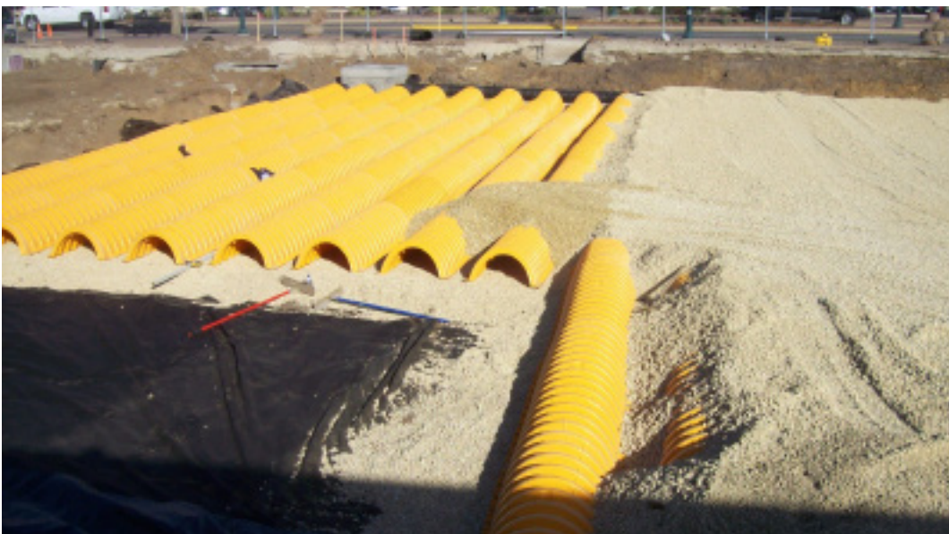
An underground detention chamber system under construction in Davenport.
