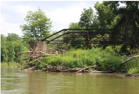
Old bridge at Hurstville Branch Creek
