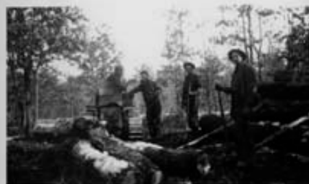
NOTE THE PILE OF LOGS
