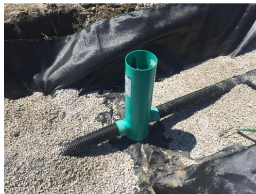
Figure C5-S4-9. Plastic catch basin with internal water level control stoplogs (see channel for stop logs inside structure)
