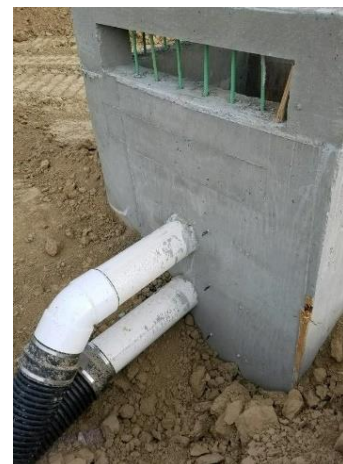
Figure C5-S4-7 A & B. Internal Water Storage subdrain with external wye for cleanout
