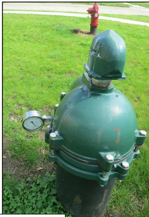
Wellhead with pressure gauge
