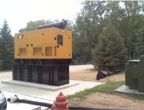
New emergency generator, to allow system to remain in operation during power outages.
