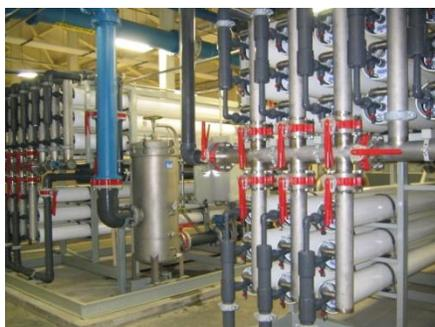
Photos from a new treatment plant with reverse osmosis filter skids (left), treatment chemicals (right), and high service pumps (below)
