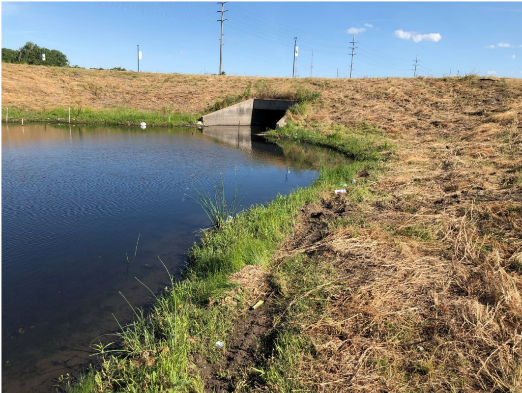
Wet forebay upstream of Gray's Station constructed stormwater wetland in Des Moines, IA.
