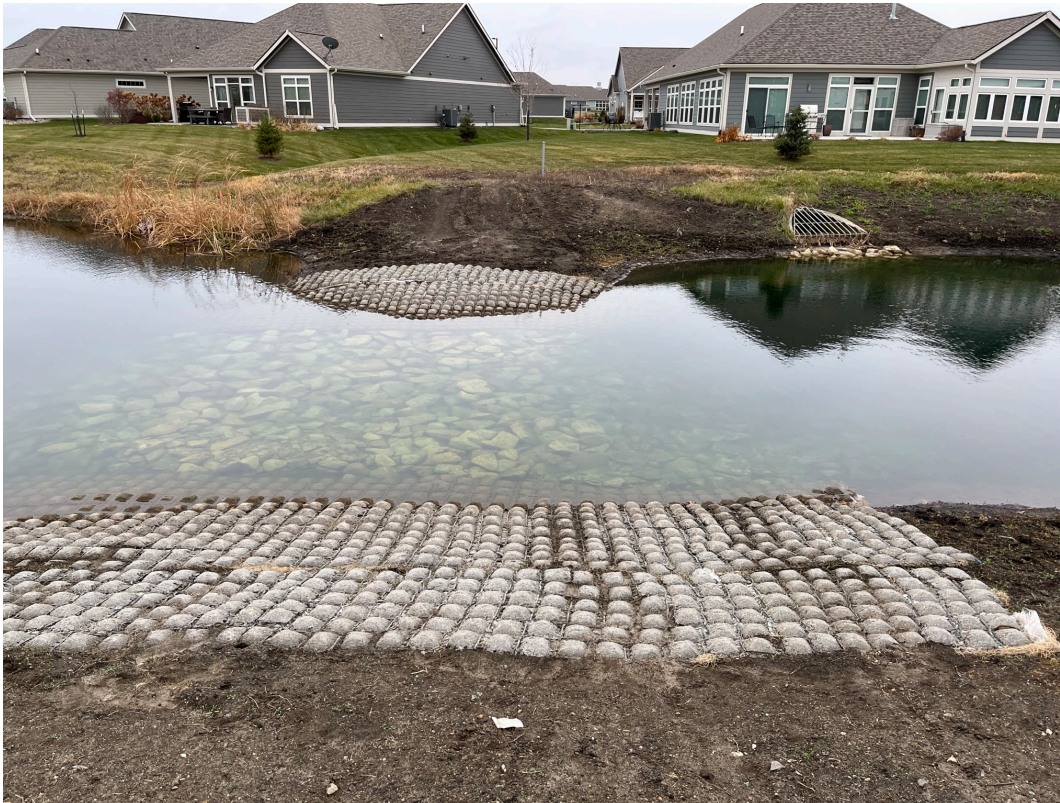
Wet forebay separated by stone embankment from downstream pond. Vegetated concrete mat used for maintenance access and scour protection at sides of stone embankment. Clive, IA.
