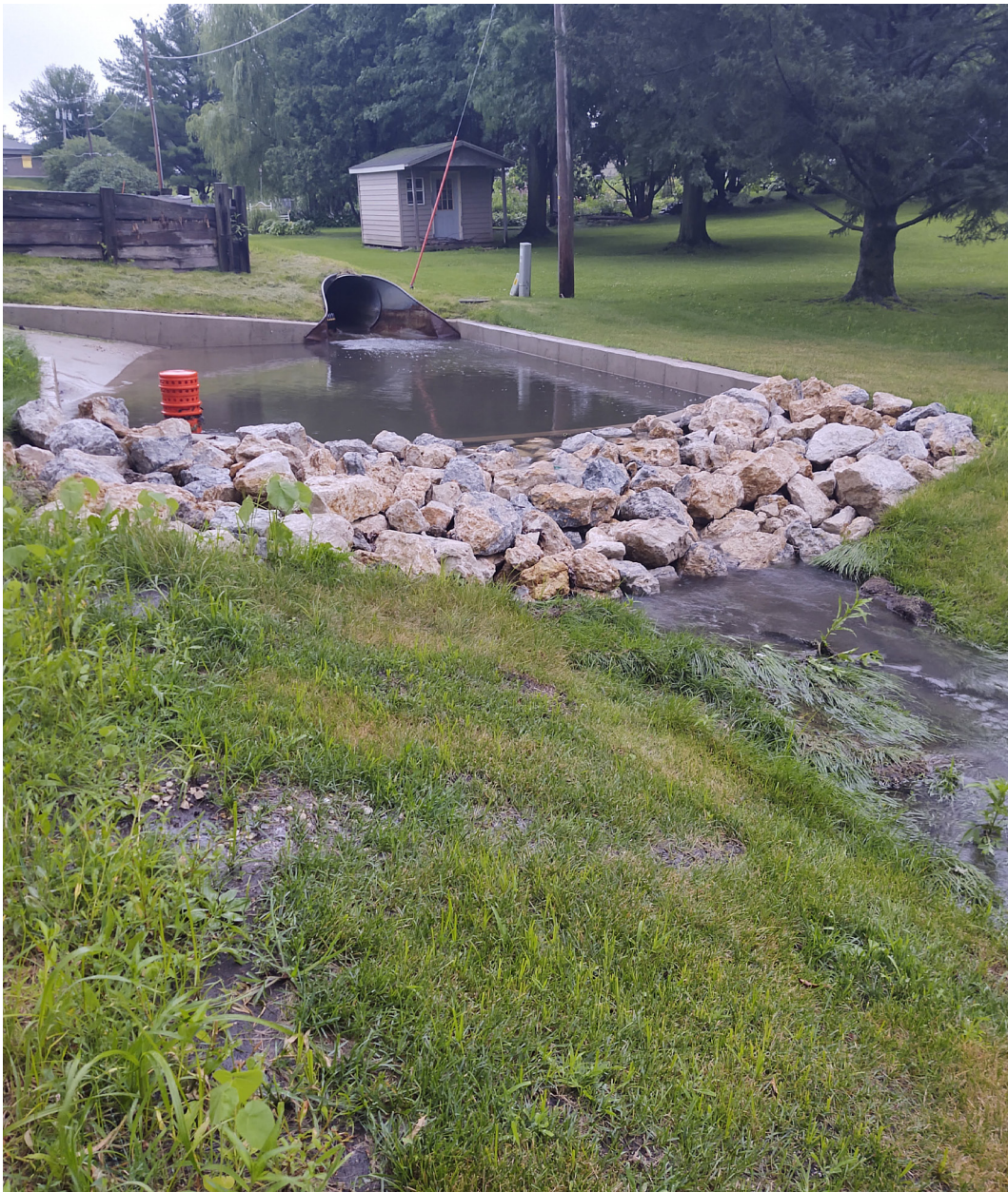
Sediment collection area upstream of a grass swale.
