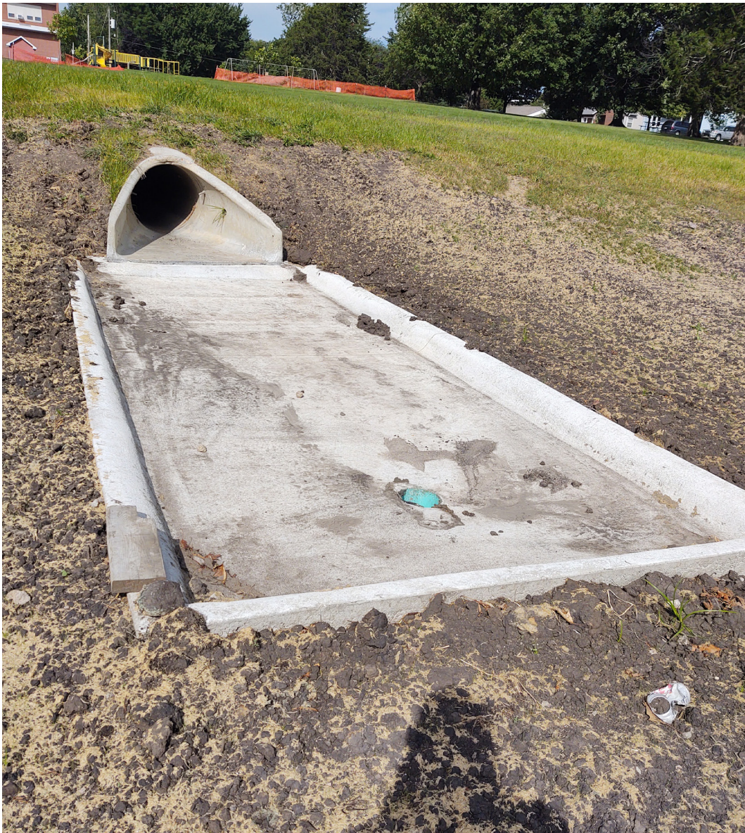
Sediment collection area just after construction.
