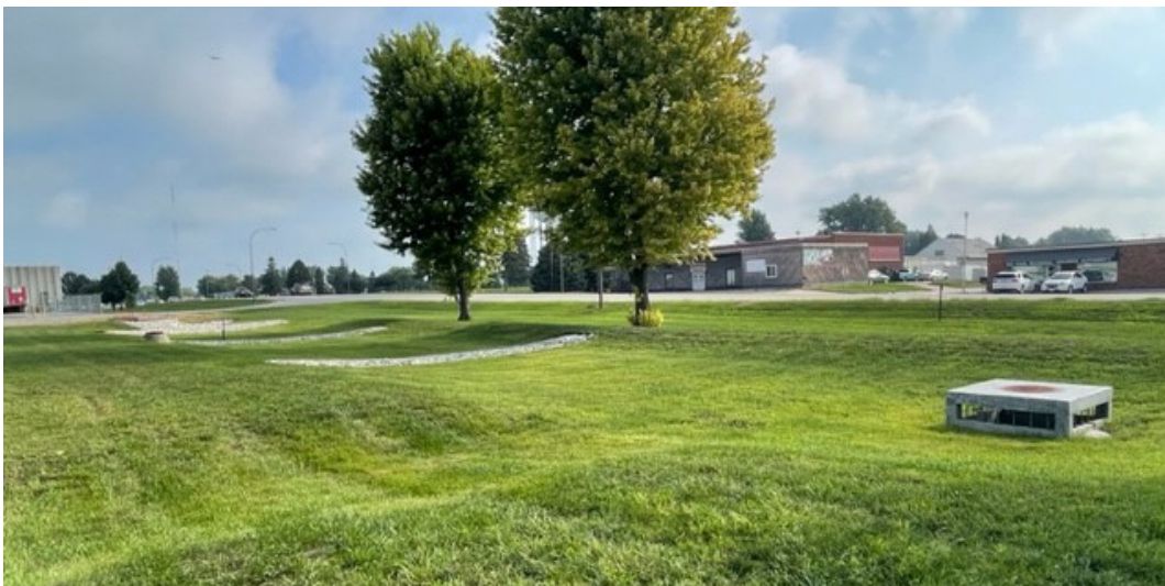
Grass swale with check dams after construction and establishment of vegetation.
