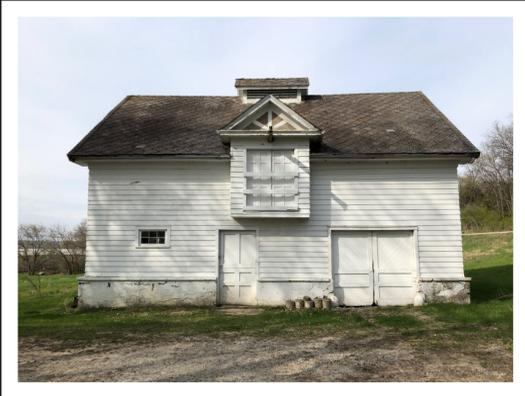
Overview of Barn in 2021, note wood siding has replaced stucco, facing west. Note: Original pebble-dash stucco can be seen in the gable between the decorative stickwork.
