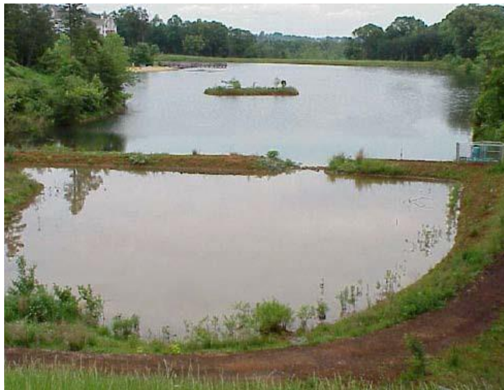
Figure C3-S11-1: Sediment forebay with earthen embankment and riprap Source: Center for Watershed Protection
