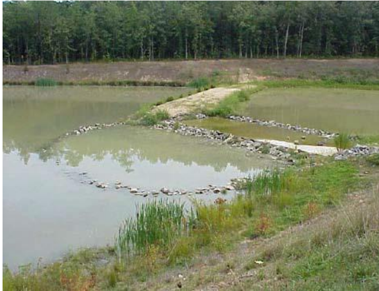
Figure C3-S11-2: Sediment forebay constructed with submerged rip-rap weir Source: Center for Watershed Protection
