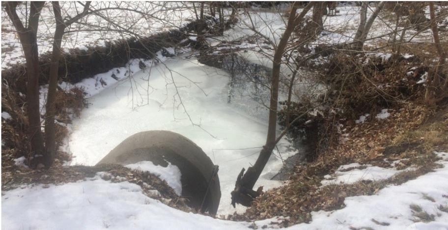
Figure 9.10-1-11-A: Level spreader outlet structure
