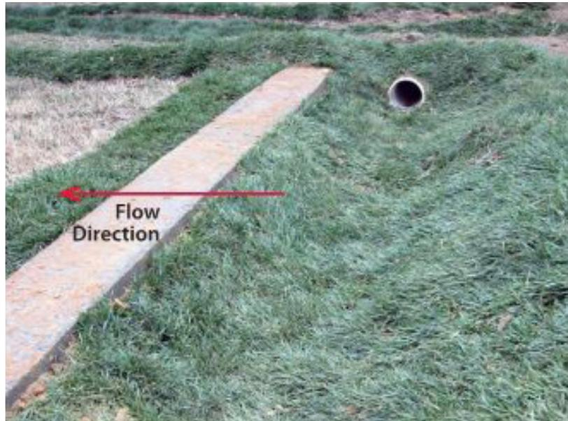
Concrete level spread with grass basin on upstream side. Flow enters from pipe that runs parallel to the spreader and leaves by filling the basin and flowing across the level concrete strip.
