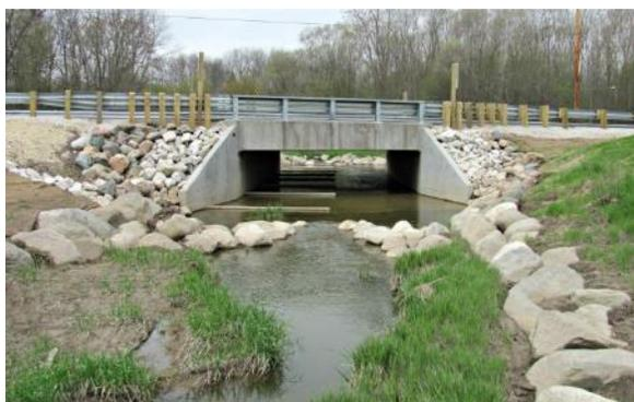
**Photo 11.** Buried concrete box culvert. Source: Ozaukee Co, WI
