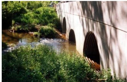
**Photo 13.** 3-culvert design with varying elevations. Maryland. Source: Delaware River Basin Commission.
