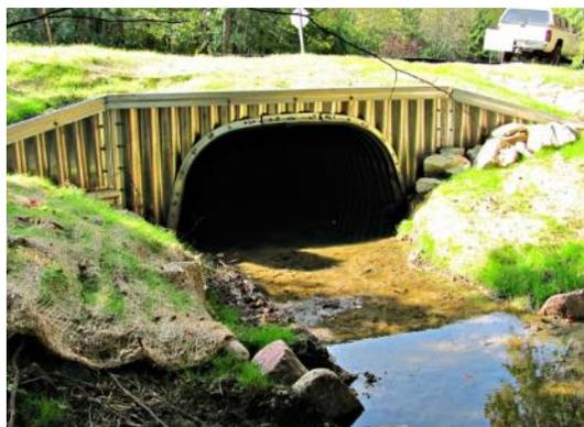
**Photo 9.** Buried aluminum box culvert. Source: Ozaukee Co, WI
