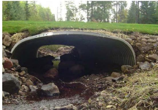
**Photo 4.** Example 2 – Mark Creek, bottomless culvert, post construction. Source: Marty Rye, Superior National Forest.
