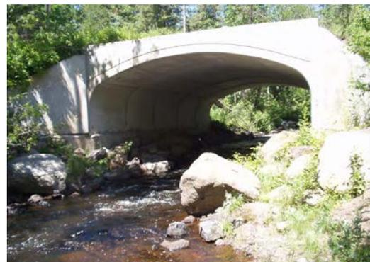
**Photo 6.** Example 3 – Tait River, bridge, 24' span, post construction. Source: Marty Rye, Superior National Forest.
