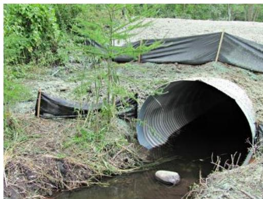
**Photo 10.** Buried aluminum circular culvert. Source: Ozaukee Co, WI
