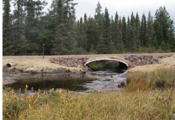
**Photo 2.** Example 1 – Inga Creek, bottomless culvert, post construction. Source: Marty Rye, Superior National Forest.
