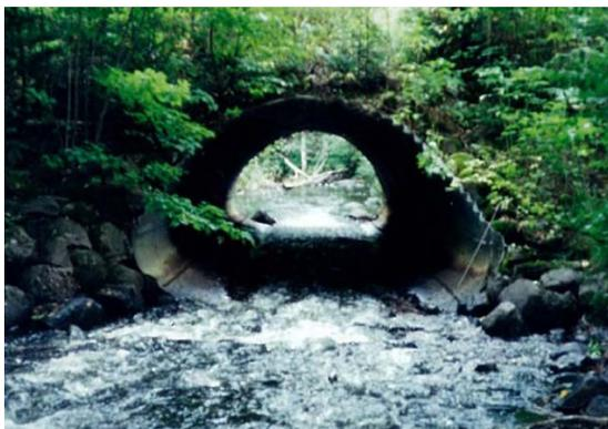
**Photo 5.** Example 3 – Tait River, culvert, 12' span, existing conditions. Source: Marty Rye, Superior National Forest.
