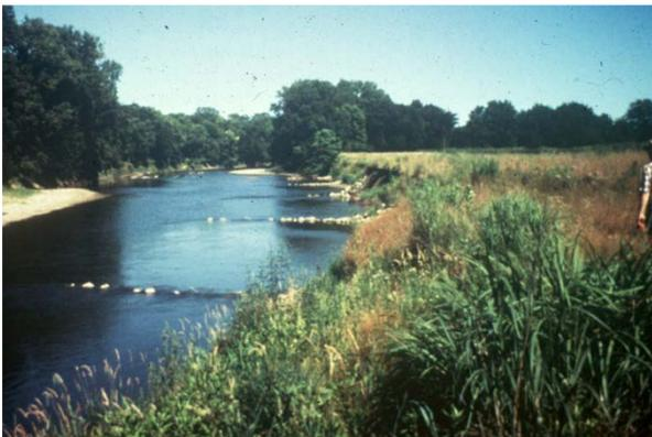
**Photo 14.** Bendway weirs visible at low flow.
