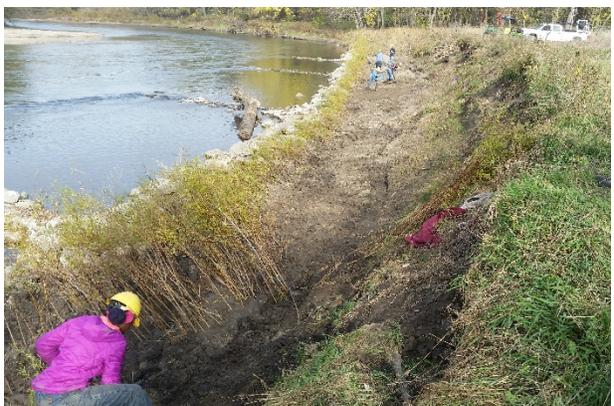
**Photo 10.** Bendway weirs and live brush layering on Boone River, Iowa. Source: Iowa DNR.
