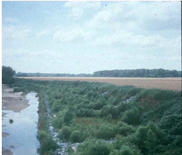
**Photo 9.** Longitudinal peaked stone toe with tie backs one year after construction; Red Banks, MS. Source: Dave Derrick
