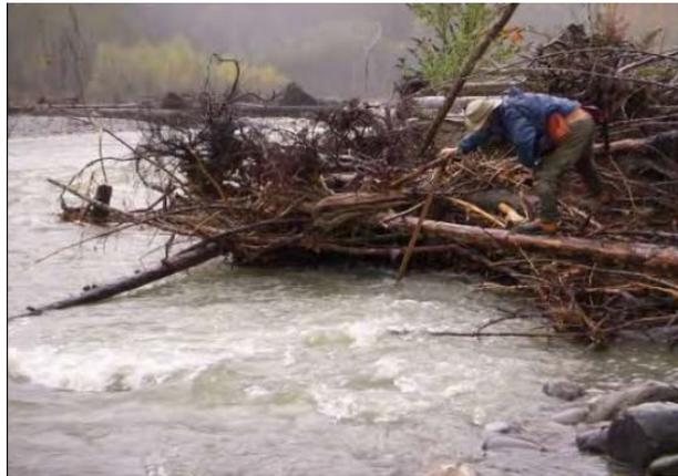
**Photo 5.** Engineered log jam on South Fork Nooksack River, Washington. Source: Southerland, 2010.
