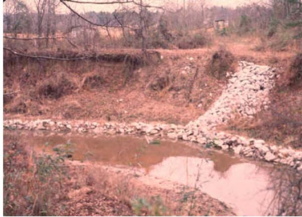
**Photo 7 .** Longitudinal peaked stone toe with tiebacks. Source: WES Handbook, USACE, 1997.
