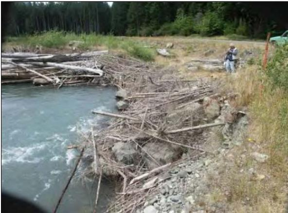
**Photo 4.** Engineered log jam on Cispus River, Washington. Source: Southerland, 2010.
