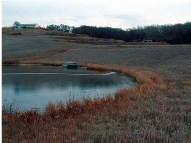
A good vegetative cover on the embankment and along the shoreline helps prevent erosion.
