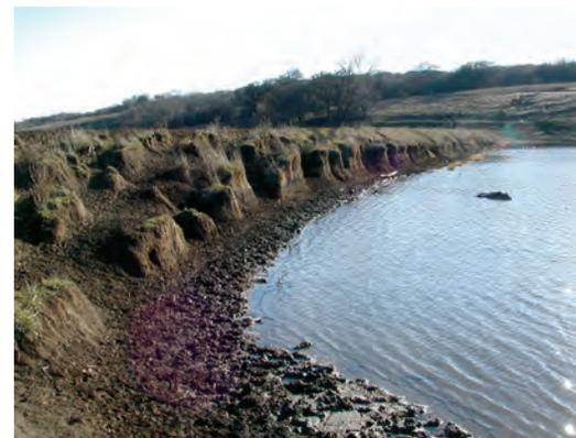
Excessive erosion on an upstream slope, due to grazing cattle and wave action.
