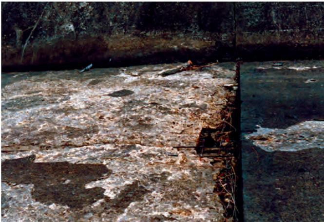
Concrete deterioration has exposed reinforcing steel and created a hole in the chute spillway floor above.
