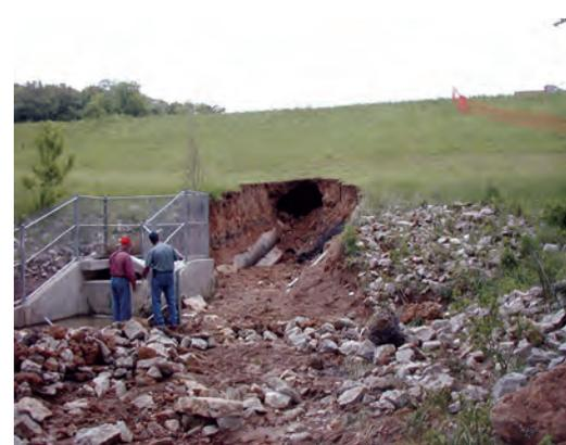
Piping failure of a dam as a result of seepage along the spillway conduit. A hole has eroded completely through the dam.
