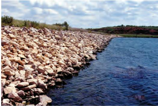
Riprap blankets protect embankments from wave erosion.
