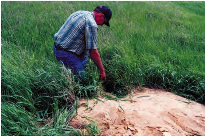
Locating a rodent burrow near an emergency spillway.
