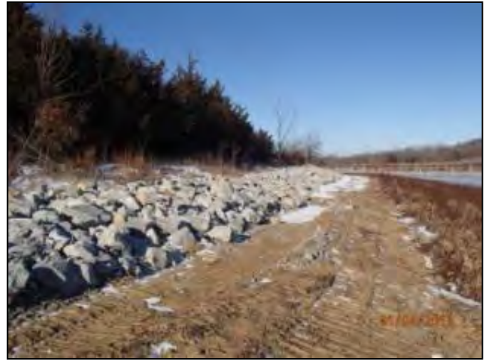
Shoreline stabilization of regions with significant erosion
