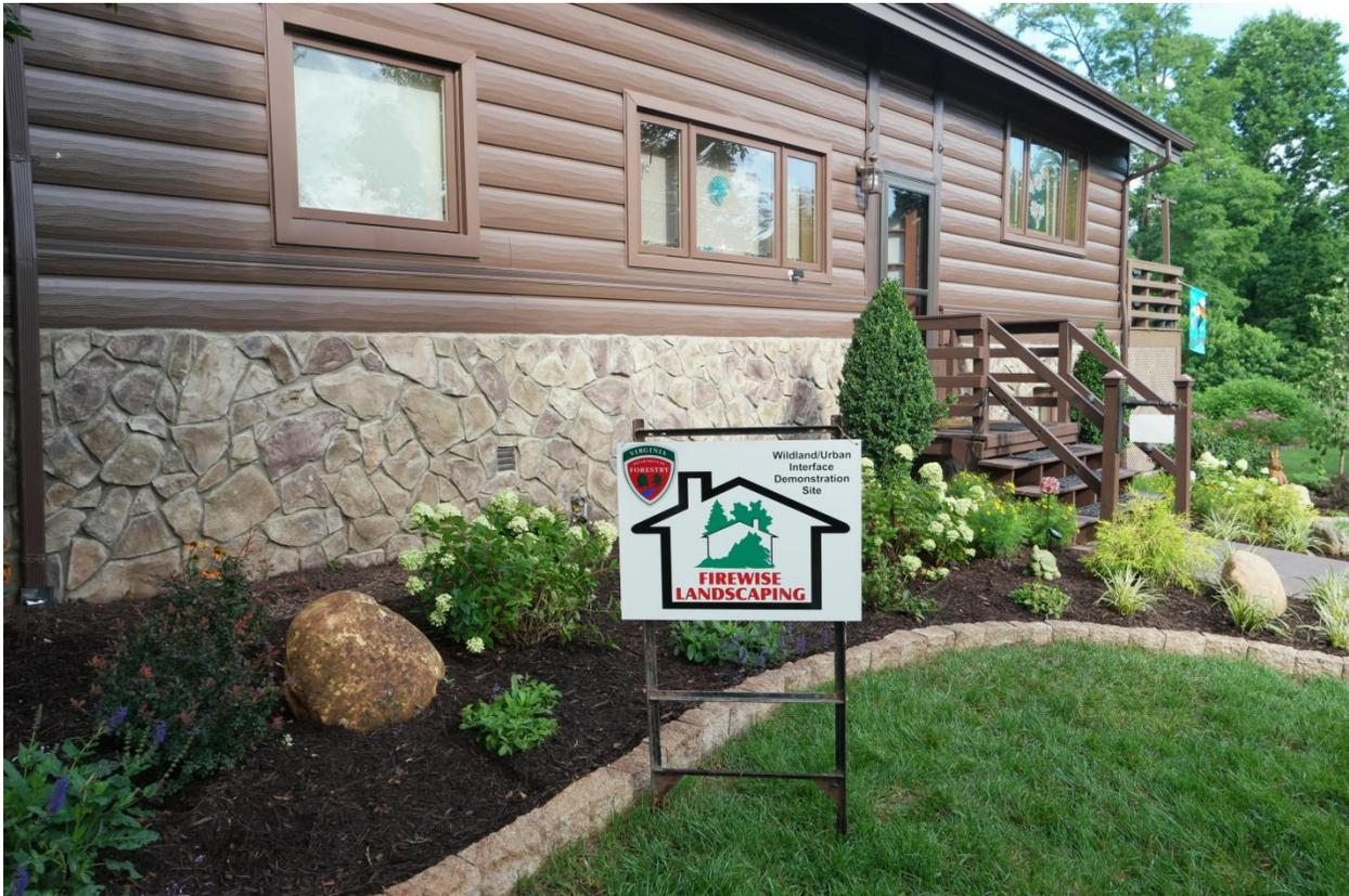
*The plants were selected for their low flammability, the foundation is rocked, and the siding is actually steel siding not real logs. Credit: Virginia Division of Forestry*
