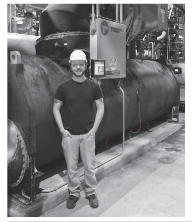
The intern focused on the buildup of scale within the chillers, caused by the hard water that is used in the system. Hard water use in a chiller system contributes to system inefficiencies and decreases it's overall capacity.
